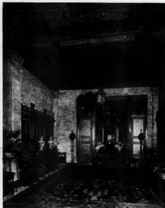
ANOTHER VIEW OF THE MAIN LOBBY OF THE PARK LANE, LOOKING TOWARD THE DINING ROOM SCHULTZE & WEAVER, ARCHITECTS
