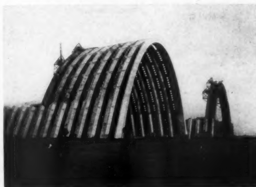
A VIEW SHOWING THE OUTER AND INNER SURFACE OF THE HANGAR AND ALSO ARRANGEMENT OF THE WINDOWS IN THE ROOF
