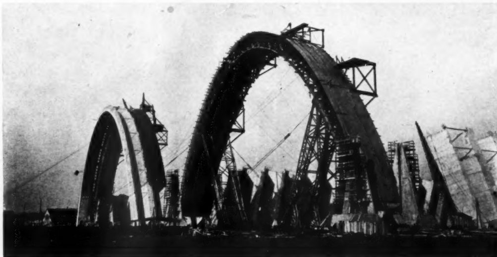
One of the wooden arched form-supports is shown at the right with its ends resting on the reinforced concrete platform truck. The ends of this arched form-support consist of a reinforced concrete beam which is moved vertically about 35'-0" by means of hydraulic jacks. The vertical guides which house the ends of this reinforced concrete girder are shown at the right lower end of the arch. In the arch shown at the left one section of concrete has been poured complete. The arched form-support has been moved to the next section, elevated in position, and the forms placed so as to complete the concrete arch. After the concrete is poured and set the outer form is removed, the arched form-support is lowered sufficiently for the lower form to clear the concrete, and it is moved forward to the next position
