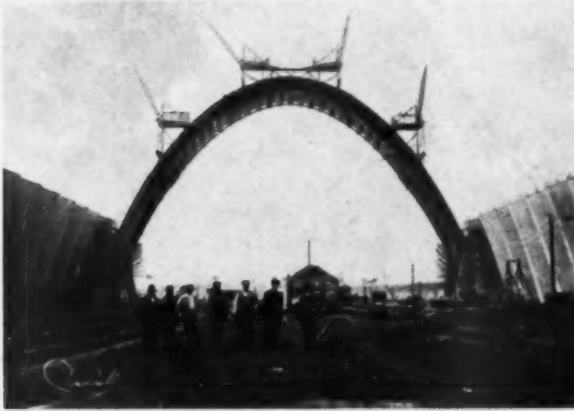
THE ARCHED FORM-SUPPORT ASSEMBLED AND SELF-SUPPORTING, READY TO BE RAISED VERTICALLY INTO ITS FINAL POSITION. THE FOUR DERRICKS ARE USED FOR PLACING THE FORMS, RAISING THE REINFORCING STEEL AND THE CONCRETE.
