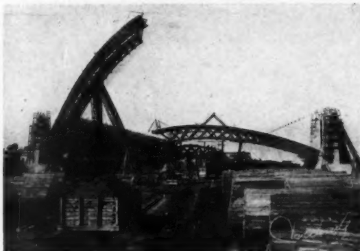
ONE SIDE OF THE LOWER SECTIONS OF THE ARCHED FORM-SUPPORT IN POSITION, THE OPPOSITE SECTION BEING RAISED AND THE CENTER, OR KEYSTONE SECTION, RESTING ON A MOVABLE TRUCK
