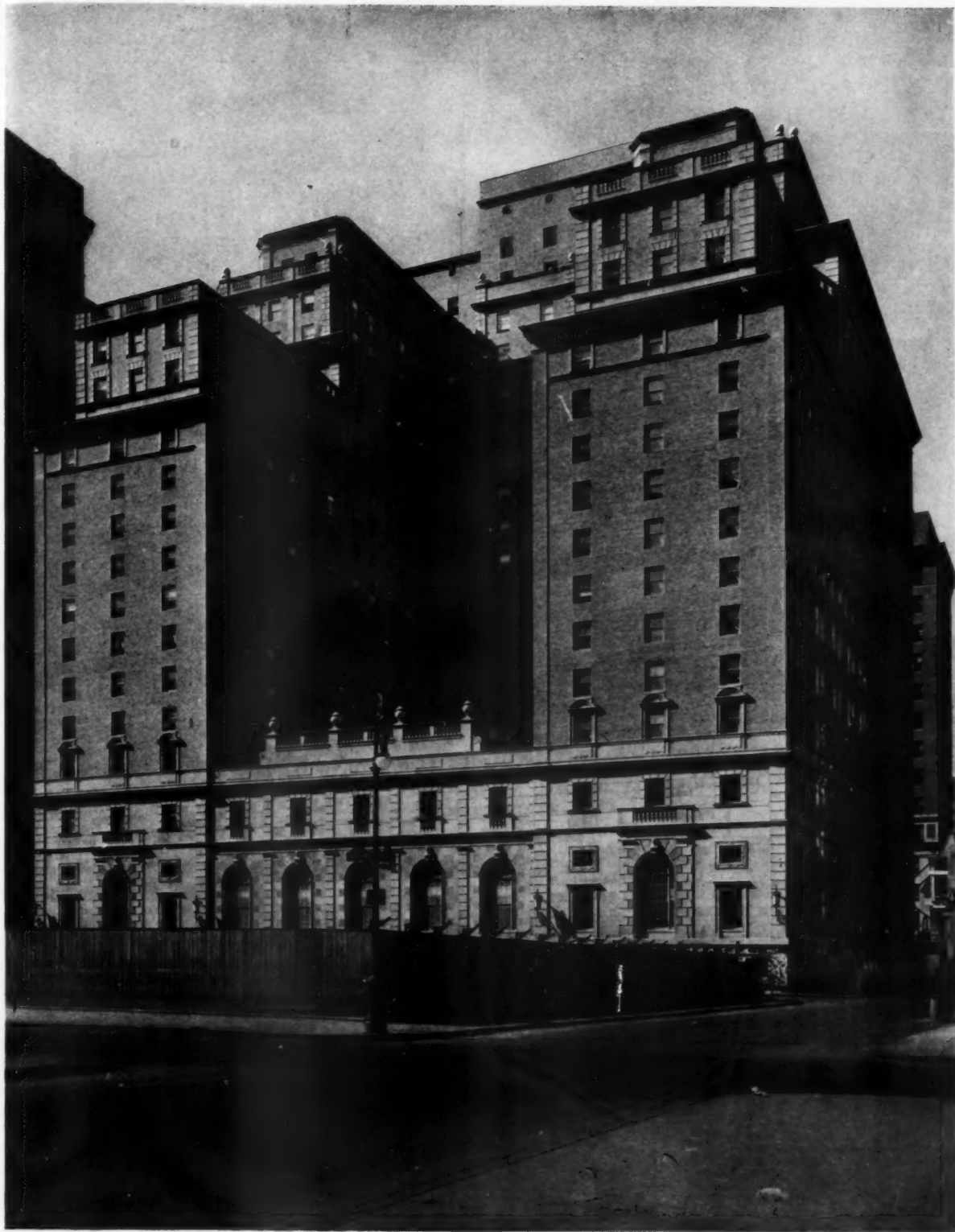
VANDERBILT AVENUE FRONT THE ROOSEVELT, NEW YORK GEORGE B. POST & SONS, ARCHITECTS
