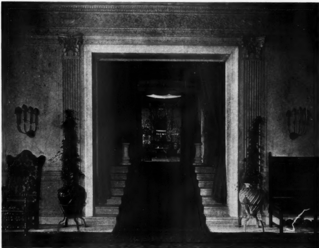
VIEW FROM LOBBY TO LOUNGE LAKE SHORE DRIVE HOTEL, CHICAGO, ILL. FUGARD & KNAPP, ARCHITECTS
