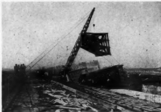
VIEW SHOWING A PORTION OF THE FOUNDATION AND A PORTION OF THE FIRST SECTION OF THE ARCH COMPLETED. THE FORMS ARE REMOVED AND RESET BY MEANS OF THE DERRICK WHICH IS ATTACHED TO THE TRUCKS
