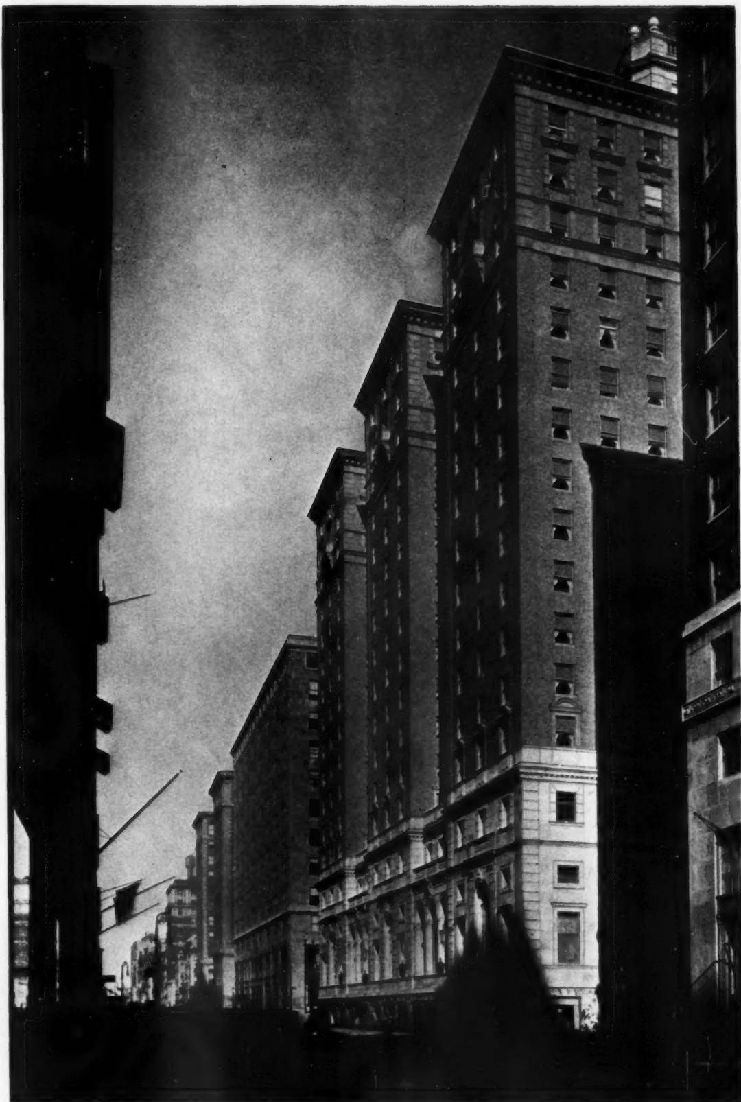
VIEW LOOKING NORTH ON MADISON AVENUE THE ROOSEVELT, NEW YORK GEORGE B. POST & SONS, ARCHITECTS
