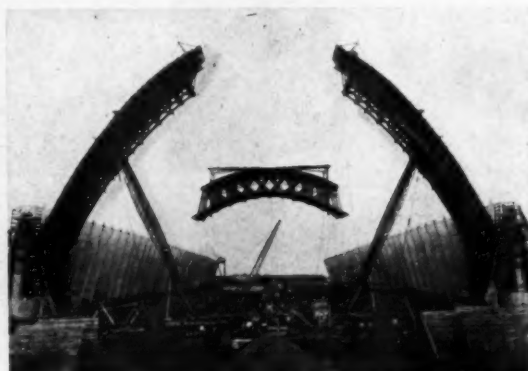
HOISTING THE CENTER OR KEYSTONE SECTION OF THE ARCHED FORM-SUPPORT INTO POSITION. THE LOWER SECTION OF THE CONCRETE ARCH ON EACH SIDE OF THE HANGAR IS COMPLETED
