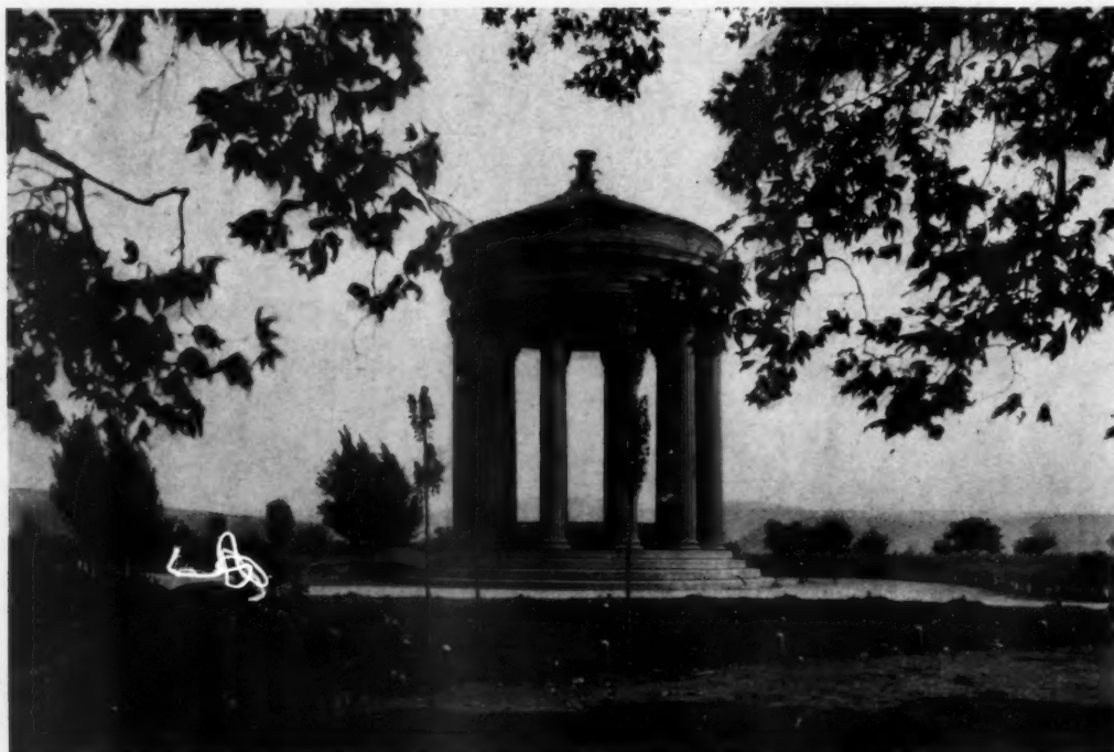
WATER TEMPLE, SUNOL, CAL., WILLIS POLK, ARCHITECT
