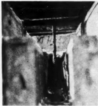
A PARAPET WALL INTO WHICH WATER ENTERED THROUGH THE VERTICAL JOINTS. THE ANCHORS WERE POORLY PAINTED AND ARE BADLY CORRODED. BUILT WITHOUT A CONSCIENCE
