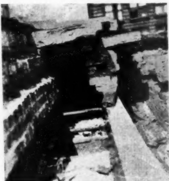
A PARAPET WALL INTO WHICH WATER ENTERED THROUGH THE VERTICAL JOINTS. THE ANCHORS WERE POORLY PAINTED AND ARE BADLY CORRODED. BUILT WITHOUT A CONSCIENCE
