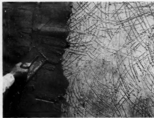
Here the finish coat is applied with the usual up and down motion but the lower or applying edge of the trowel is allowed to move in and out in an irregular way so that the stucco is thicker in some places than in others
