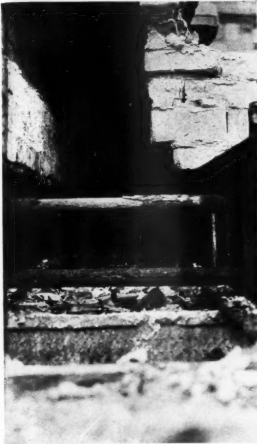
POORLY PAINTED ANCHORS ARE MUCH CORRODED BY THE WATER WHICH CAME THROUGH THE VERTICAL JOINTS
