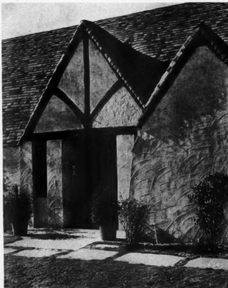
The finished result as shown in the accompanying "progress pictures." This surface adds the proper effect to the shingles and half timbering
