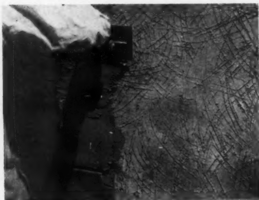
Here the finish coat is applied with the usual up and down motion but the lower or applying edge of the trowel is allowed to move in and out in an irregular way so that the stucco is thicker in some places than in others
