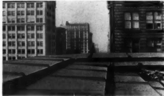
THE DISINTEGRATION OF THE WALL IS VERY APPARENT. THE WATER ENTERED THROUGH THE VERTICAL JOINTS. WHEN THE CORNICE WAS OPENED UP IT WAS FULL OF MOISTURE AND CONTAINED SOME FOUL WATER
