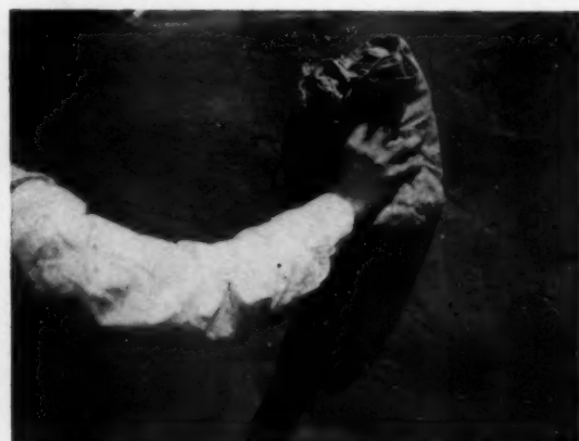
While it is still soft the sharper breaks in the mortar are worked down with the end of the trowel. About an hour after the finish is applied it is vigorously rubbed with a burlap bag which removes practically all of the trowel marks, leaving a granular, sandy surface
