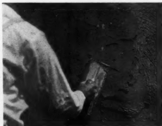
While it is still soft the sharper breaks in the mortar are worked down with the end of the trowel. About an hour after the finish is applied it is vigorously rubbed with a burlap bag which removes practically all of the trowel marks, leaving a granular, sandy surface
