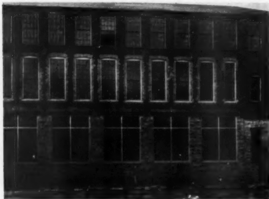
FIGURE 1. THE FIRST FLOOR OF THIS OLD BUILDING WAS REMODELLED, RESULTING IN 150% MORE DAYLIGHT FOR 63% INCREASED WINDOW AREA. AT THE EXTREME RIGHT MAY BE SEEN ONE OF THE ORIGINAL WINDOWS
