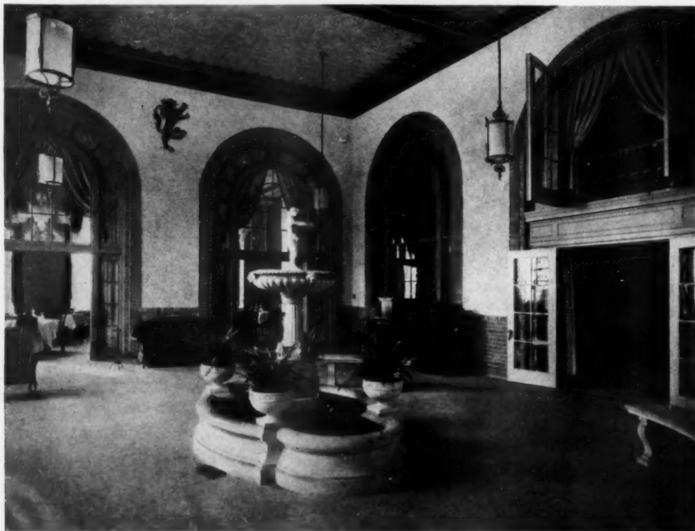
FOUNTAIN ROOM, NEW BETHLEHEM HOTEL
