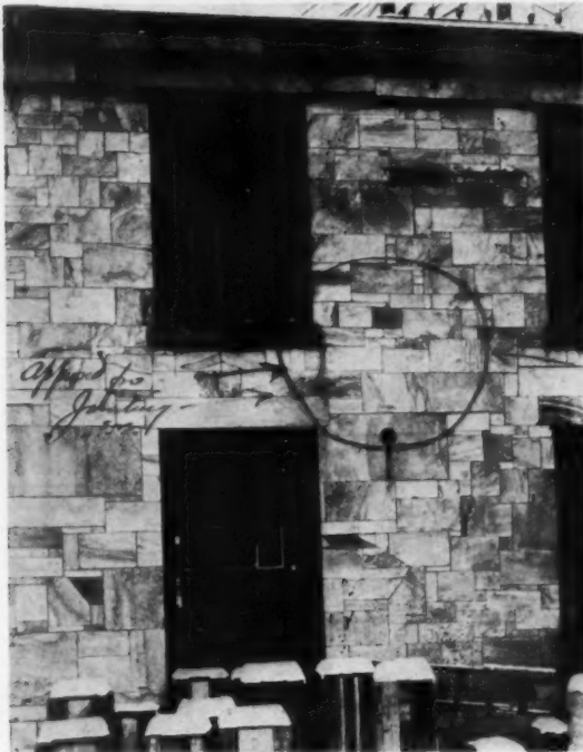
SECTION OF AN OLD MARBLE WALL, MARKED AS AN APPROVED SAMPLE OF JOINTING
