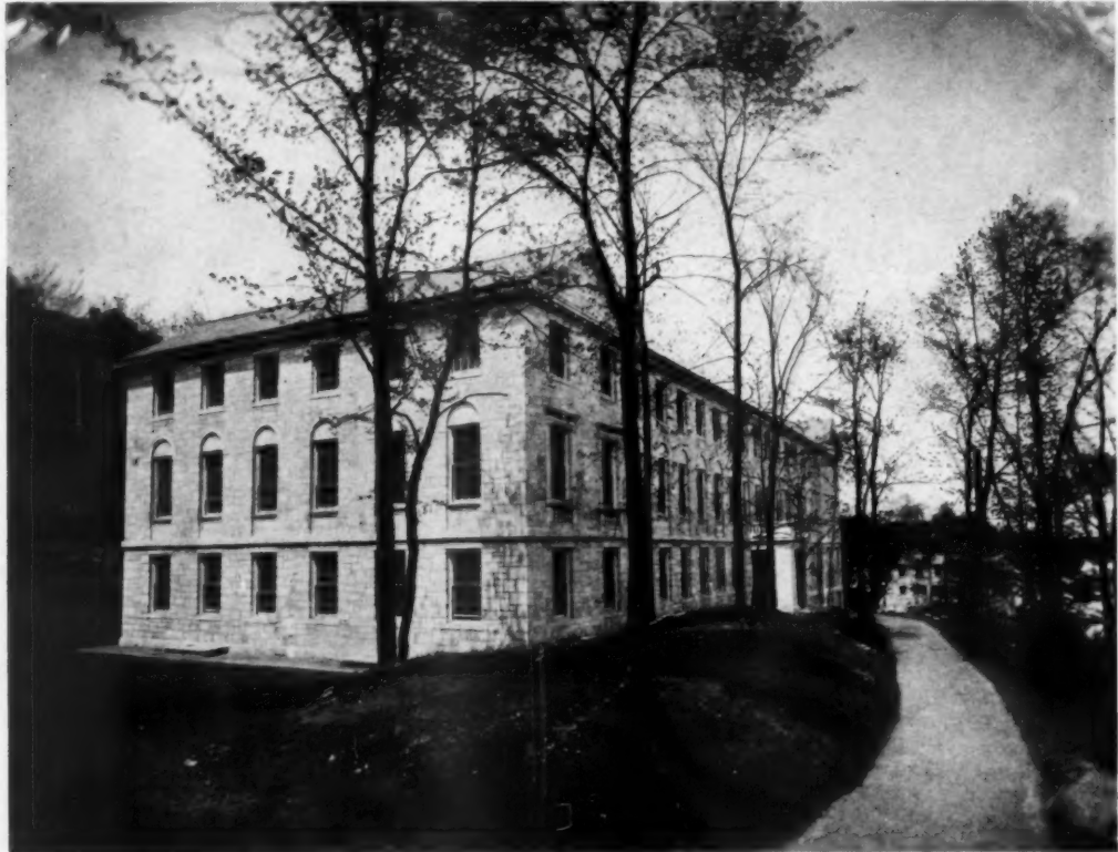
THE SOUTH FRONT SHOWS THE MARBLE ASHLAR, THE COST OF WHICH RUNS ONLY A LITTLE ABOVE THAT OF GOOD BRICKWORK
