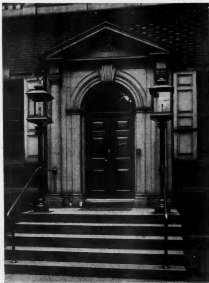
DETAIL OF NORTH ENTRANCE
