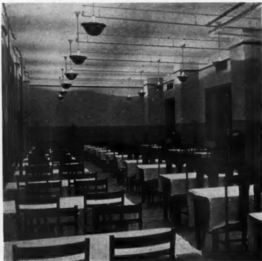
Soft, well diffused illumination is provided in this industrial dining room from 100 watt clear Mazda C lamps in mirrored glass totally indirect luminaires of simple design. Outlets are placed 10'-0" on centers
