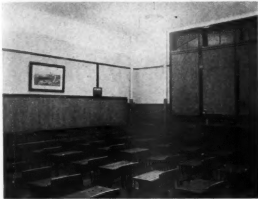
A uniform distribution of well diffused light is provided in this school room from five 200 watt Mazda C lamps in metal and glass semi-indirect luminaires. Lighting of this kind preserves the vision of the pupil and is desirable
