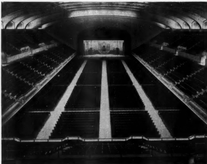
THE EVENNESS OF LIGHT DISTRIBUTION THROUGHOUT THE CLEVELAND PUBLIC HALL IS PARTICULARLY NOTICEABLE. THIS EFFECT IS SECURED BY THE ARRANGEMENT OF THE LIGHTING UNITS IN THE ATTIC
