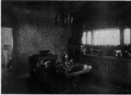
A convenience outlet in the center of the dining room serves the table appliances. A duplex outlet on the buffet operates the fan, percolator, chafing dish, lamp or other device. A heating outlet is in the baseboard
