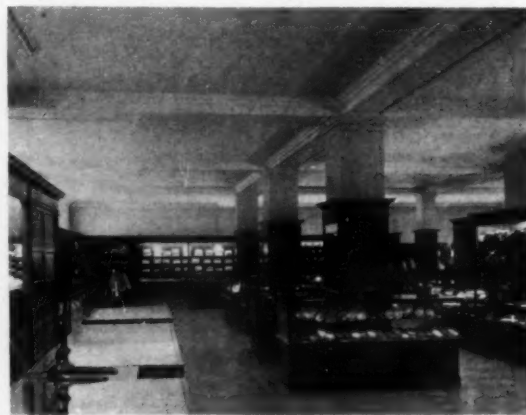
EFFECTIVE INSTALLATION OF INDIRECT LIGHTING FOR GENERAL ILLUMINATION IN A LARGE MEN'S FURNISHING STORE, WITH DIRECT LOCAL LIGHTING IN THE SHOW CASES
