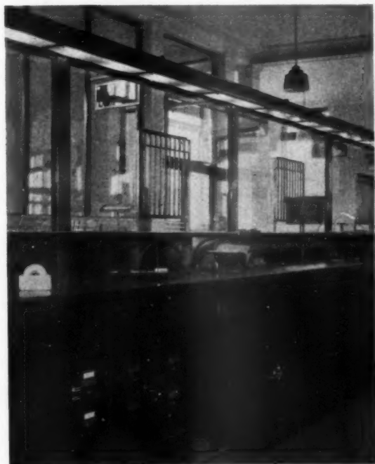
DIRECT LIGHTING SYSTEM TO ILLUMINATE THE WORKING SPACE IN A BANK
