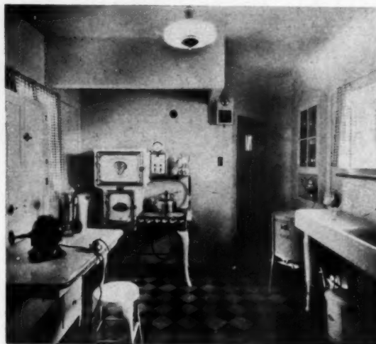
The kitchen has a power outlet for the electric range. Duplex outlets for mixers, utility motor, fan and other appliances
