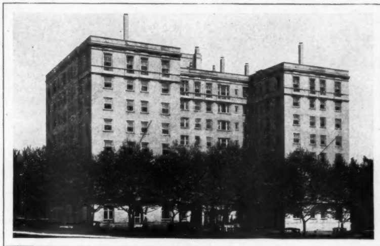
RUSKIN APARTMENTS, Pittsburgh, Pa.: H. L. Steens & Company, New York, Architects; Bailey-Farrel Mfg. Co., Pittsburgh, Jobbers; Wey Bros., Pittsburgh, Plumbers
