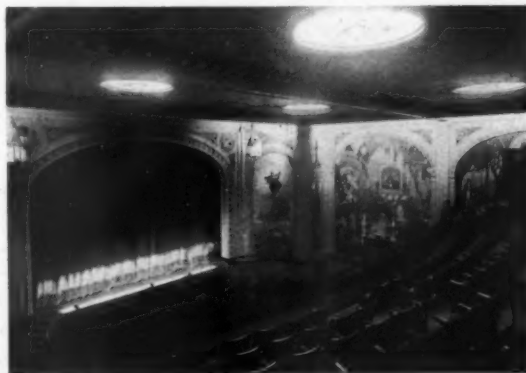
The decorative element is very important in the lighting of ornamental interiors, such as theatres. In this particular installation general illumination is provided from lamps placed above circular openings in the ceiling, filled with decorated diffusing glass. The highly colored mural paintings are especially lighted by lamps in angle reflectors concealed from view. In each side of the proscenium arch is hanging a castle of colored glass made luminous by lamps placed therein. Standard equipment is unsuitable for such work
