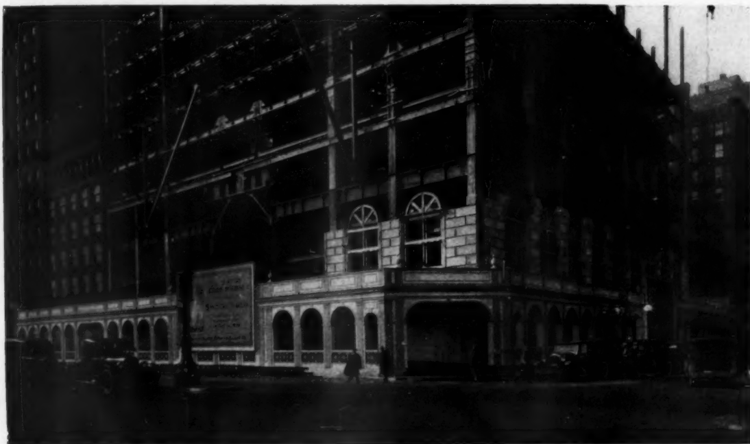
SIDEWALK PROTECTION, STRAUS BUILDING, CHICAGO, ILL. GRAHAM, ANDERSON, PROBST & WHITE, ARCHITECTS
