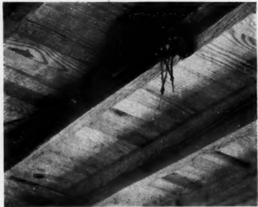
ARMORED CABLE. WIRING TO COMBINATION FIXTURE IN KITCHEN CEILING
