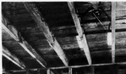
ARMORED CABLE. WIRING IN LIVING ROOM CEILING, FIRST FLOOR
