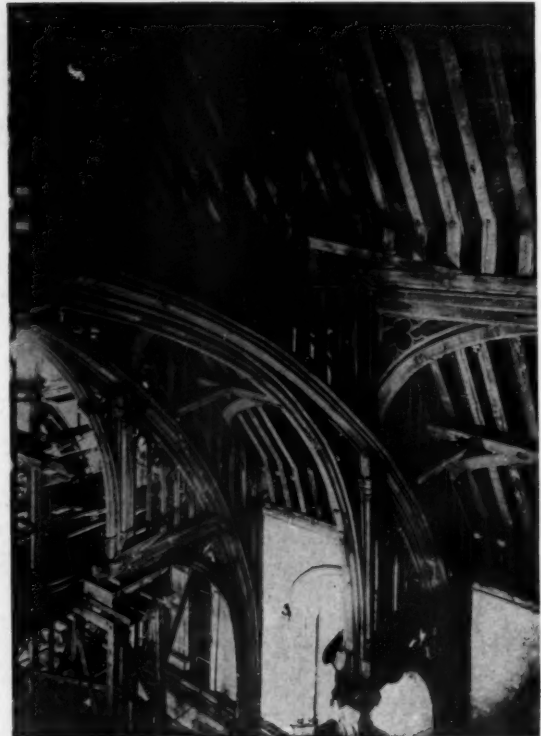
VIEW TAKEN FROM LEVEL OF GREAT COLLAR AND TRUSSED PURLIN BEFORE RECENTLY EXECUTED REPAIRS
