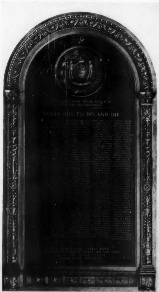
MEMORIAL TABLET, LARGE PYLON, WASHINGTON MEMORIAL BRIDGE
