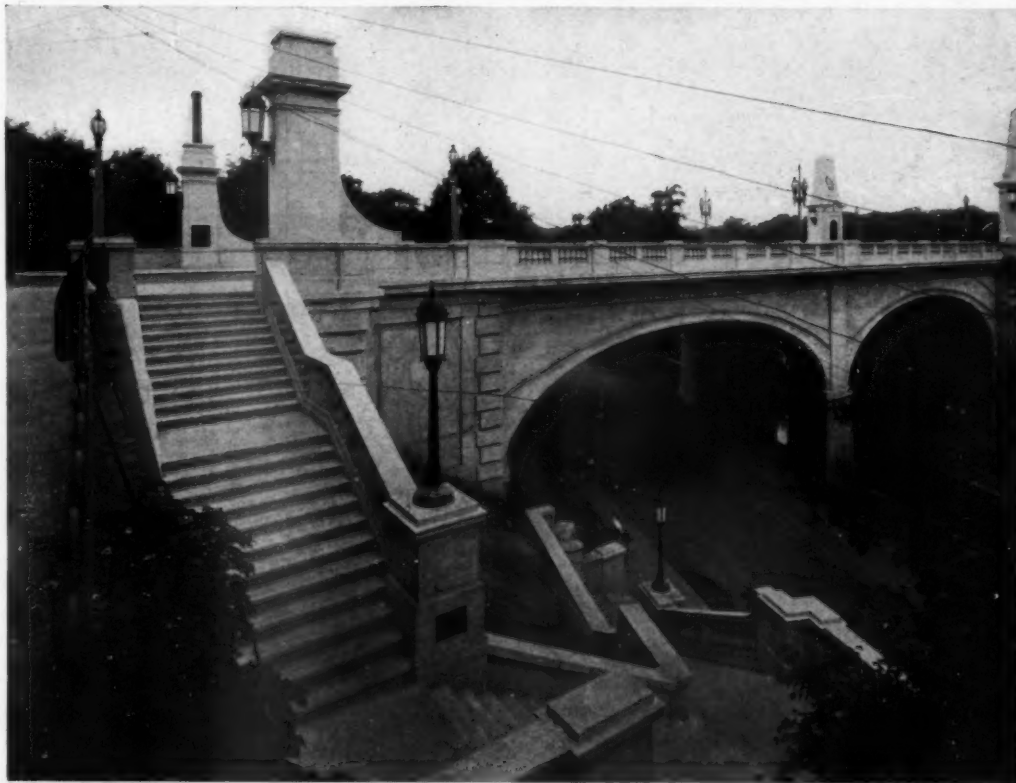
WASHINGTON MEMORIAL BRIDGE, WILMINGTON, DEL. VANCE W. TORBERT, ARCHITECT—BENJAMIN H. DAVIS, ENGINEER
