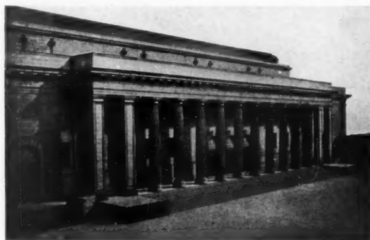
SOUTH FRONT CAIRD HALL, DUNDEE JAMES THOMSON, F. R. I. B. A., CITY ARCHITECT
