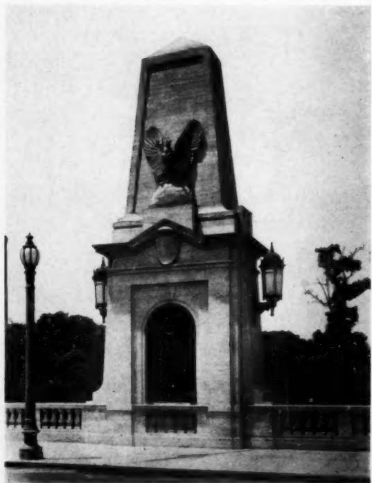
LARGE PYLON, WASHINGTON MEMORIAL BRIDGE
