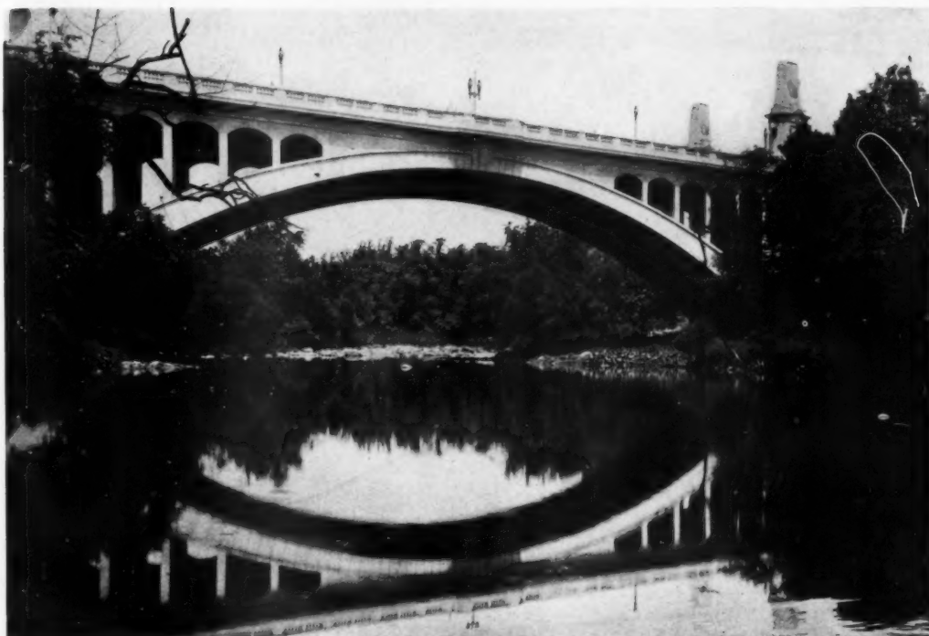
WASHINGTON MEMORIAL BRIDGE, WILMINGTON, DEL. VANCE W. TORBERT, ARCHITECT—BENJAMIN H. DAVIS, ENGINEER
