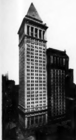
Bankers Trust Co., New York, N. Y. Arch.: Chas. I. Birge. Con't: R. H. MacDonald. Rfr.: Tuttle Roofing Co. All of New York City.
