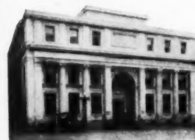
Birmingham Trust & Savings Bank, Birmingham, Ala. Arch.: Miller & Martin. Con't: Day & Sachs. Rfr.: George F. Wheelock Co. All of Birmingham, Ala.
