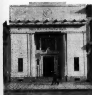
National Exchange Bank, Augusta, Ga. Arch.: Mowbray & Uffinger, New York, N. Y. Con't: Southern Ferro-Concrete Co., Atlanta, Ga. Rfr.: C. P. Murphy's Sons, Atlanta, Ga.
