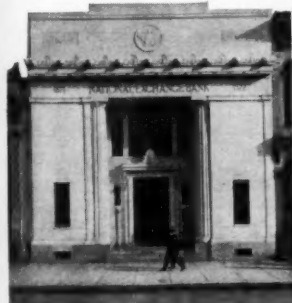
National Exchange Bank, Augusta, Ga. Arch.: Mosbray & Uffinger, New York, N. Y. Con't: Southern Ferro-Concrete Co., Atlanta, Ga. Rfr.: C. P. Murphy's Sons, Atlanta, Ga.
