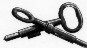
EXAMPLE OF ONE OF THE FIRST TUBULAR CYLINDER LOCKS MANUFACTURED. REPRODUCED FROM A WOOD-CUT IN A CATALOG OF BUILDERS' HARDWARE IN 1876
