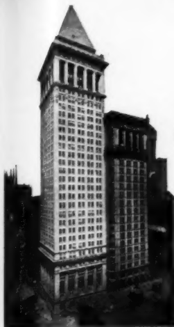
Bankers Trust Co., New York, N. Y. Arch.: Chas. I. Birge. Con't: R. H. MacDonald. Rfr.: Tuttle Roofing Co. All of New York City.
