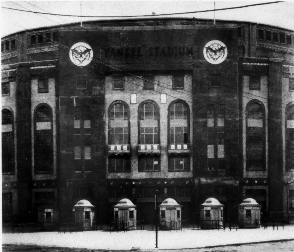
FIG. 2. MAIN ENTRANCE, YANKEE STADIUM, NEW YORK
