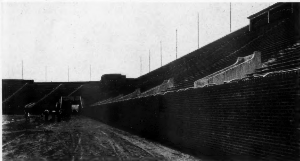
INTERIOR VIEW, FRANKLIN FIELD STADIUM, UNIVERSITY OF PENNSYLVANIA
