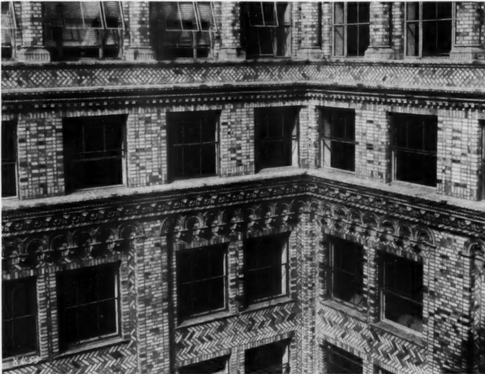
Brick and terra cotta detail at twentieth story level Pershing Square Building, New York York & Sawyer and John Sloan, Architects
