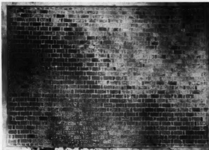
Fig. 11. Exposed side of 8" hollow restrained Western surface clay brick wall after 6-hour fire test, Test No. 5
