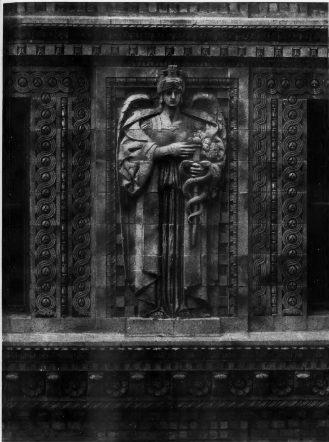
TERRA COTTA PANEL AND DETAIL AT FIFTH STORY LEVEL PERSHING SQUARE BUILDING, NEW YORK YORK & SAWYER AND JOHN SLOAN, ARCHITECTS
