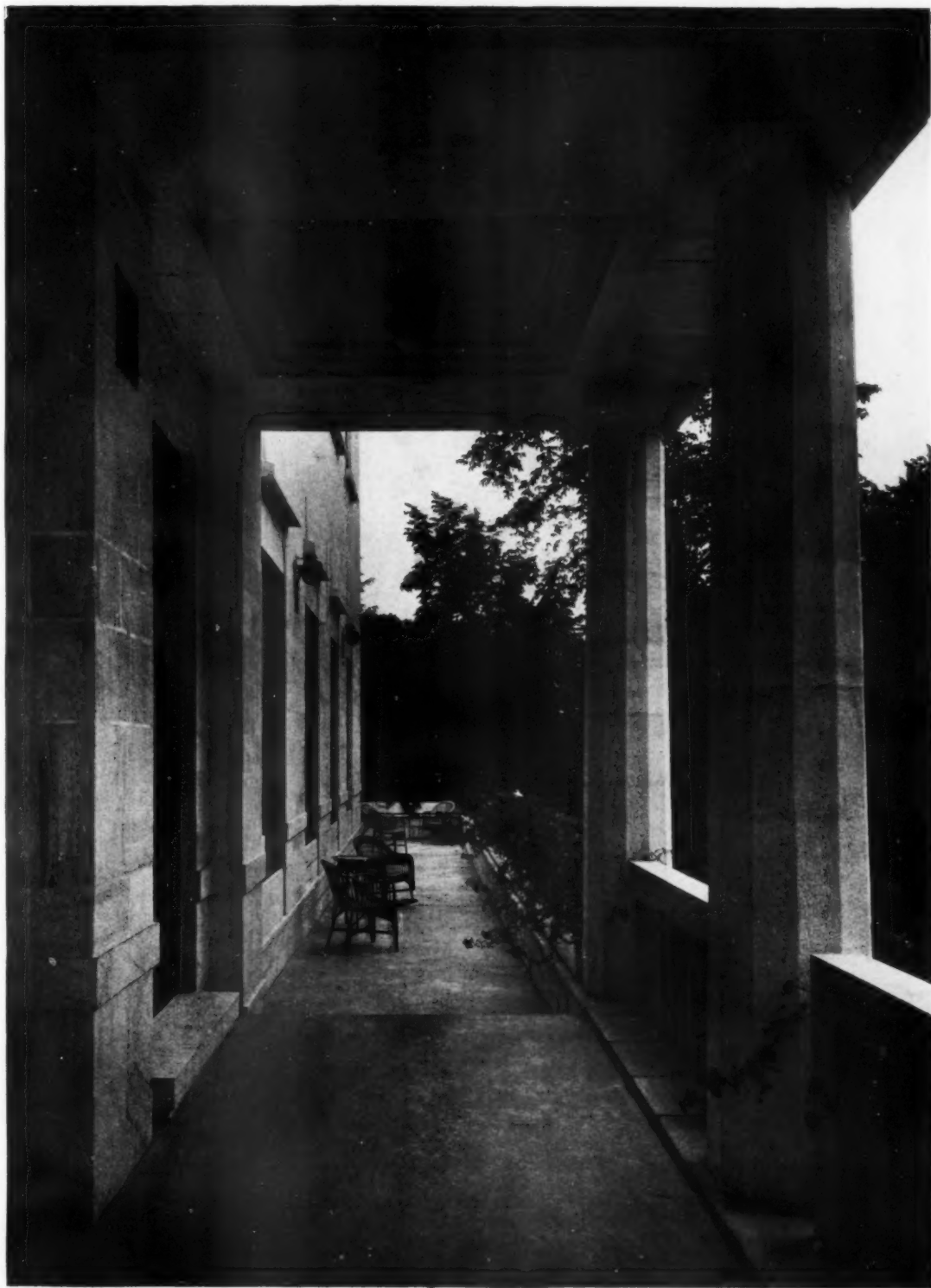
TERRACE, VILLA KEIRKNER, HELSINGFORS, FINLAND ELIEL SAARINEN, ARCHITECT
