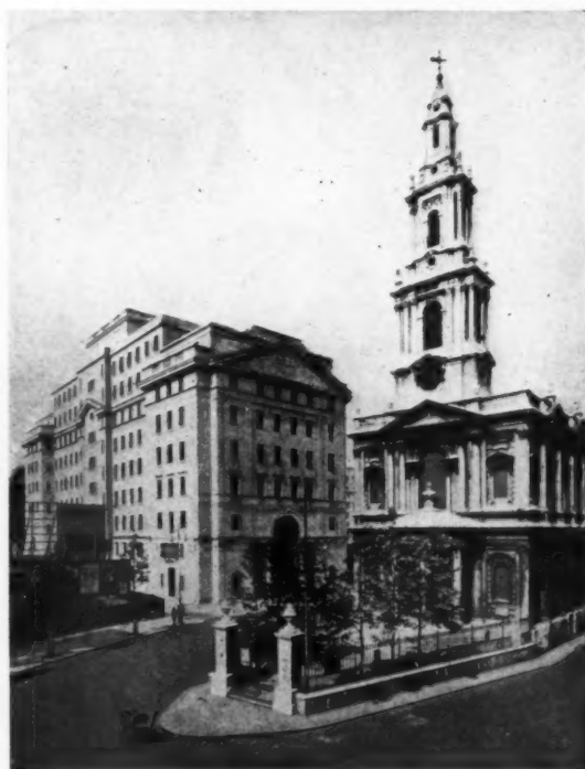
Bush House, London Helmie & Corbett, Architects
