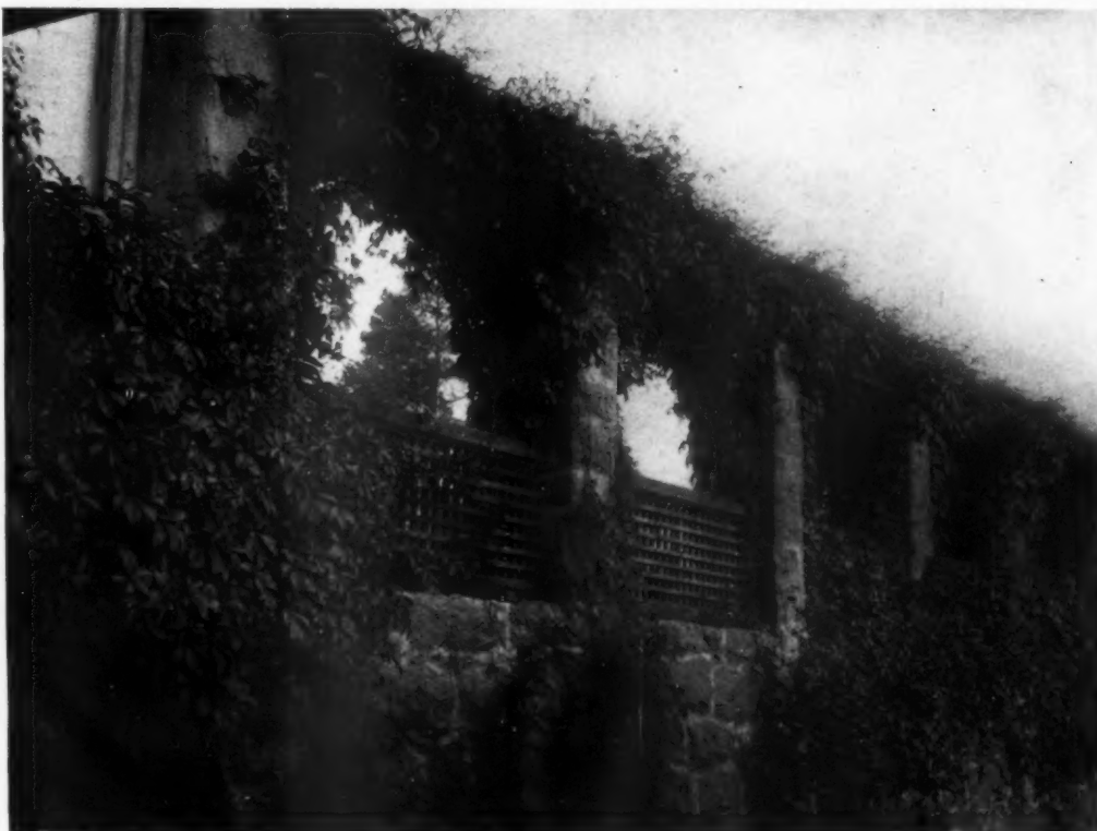
TERRACE, HOUSE OF ELIEL SAARINEN, ARCHITECT ELIEL SAARINEN, ARCHITECT
