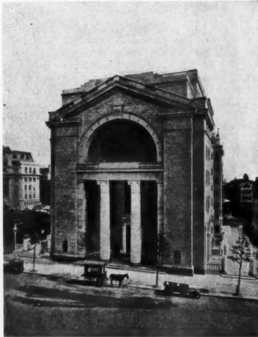
Bush House, London, view looking South Helmle & Corbett, Architects
