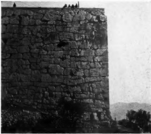
Alatri, Italy Etruscan Masonry—Pre-Roman
