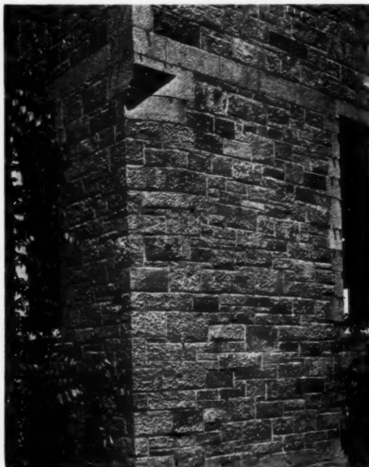
New Building, McGill University, Montreal, Canada Squared gray limestone Rubble roughly dressed—Modern
