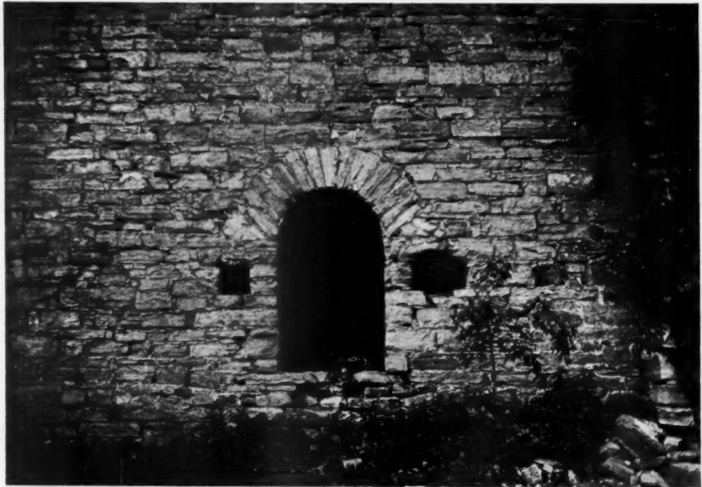
Old Mill, Chateauguay, Province of Quebec, Canada Rubble, with natural square cleavage (red and brown)—Early Eighteenth Century
