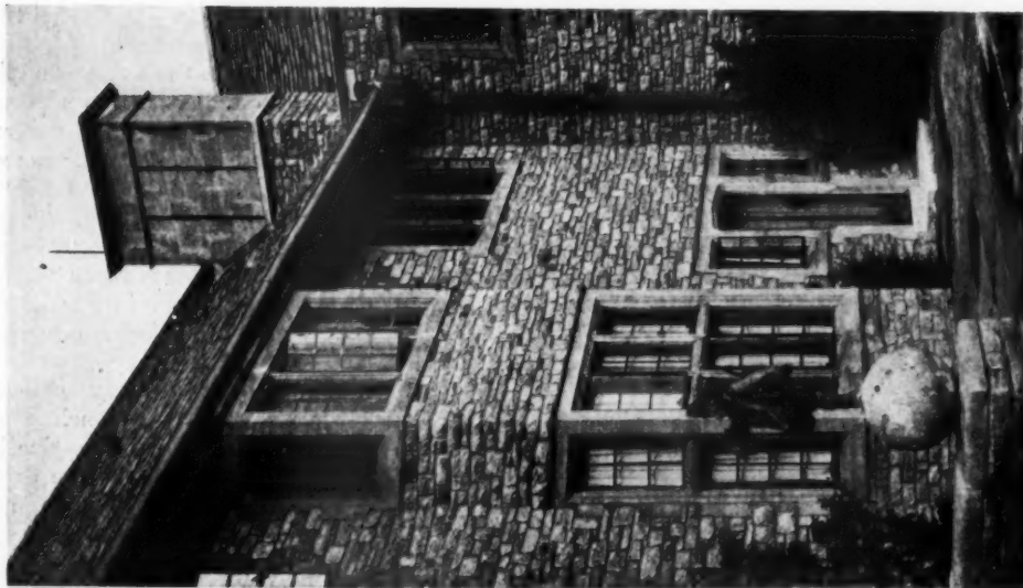
Wallingford, England Roughly squared limestone Rubble with uneven beds—Modern
