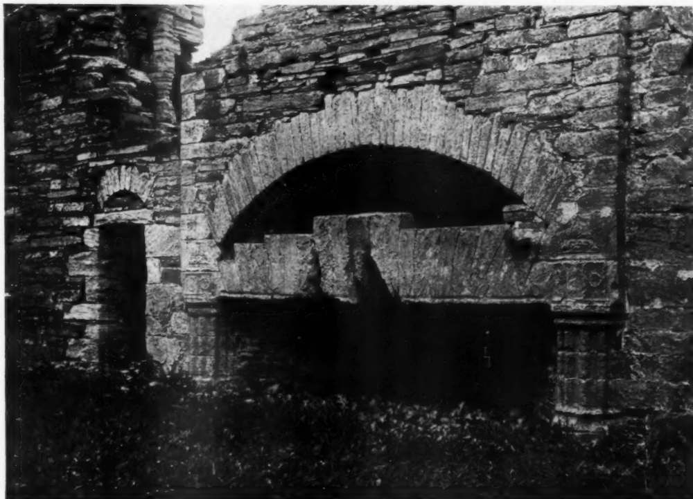
Earl's Palace, Kirkwall, Scotland Ashlar merged with Rubble of horizontal texture—Fifteenth Century
