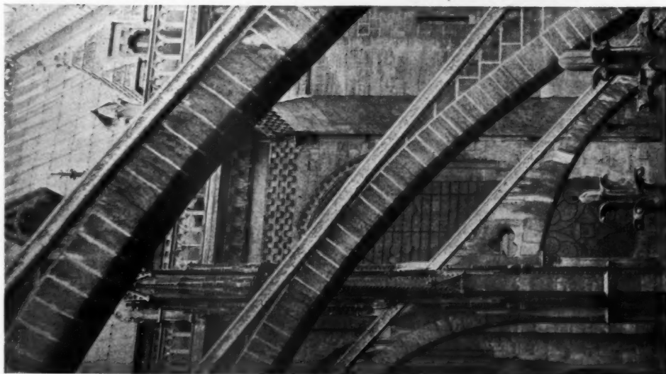
Flying Buttresses, Notre Dame, Paris— Thirteenth Century Marked jointing gives emphasis to form
