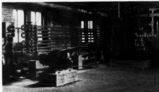
Refrigerating Plant, with Compressor, Condenser, Receiver and Electric Cabinet
