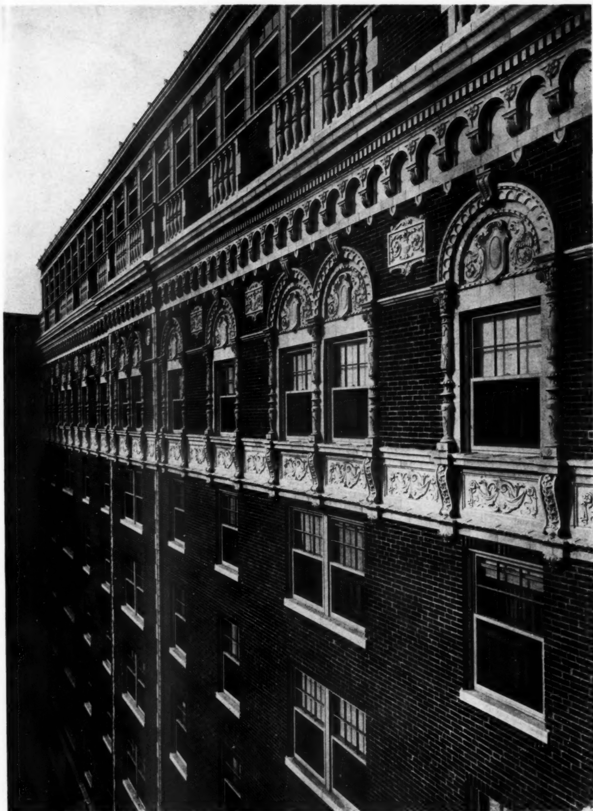
DETAIL OF UPPER STORIES THE CHASE HOTEL, ST. LOUIS, MO. PRESTON J. BRADSHAW, ARCHITECT
