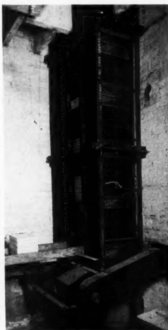
Bottom of a Subveyor Before the Enclosing Partition is Installed
