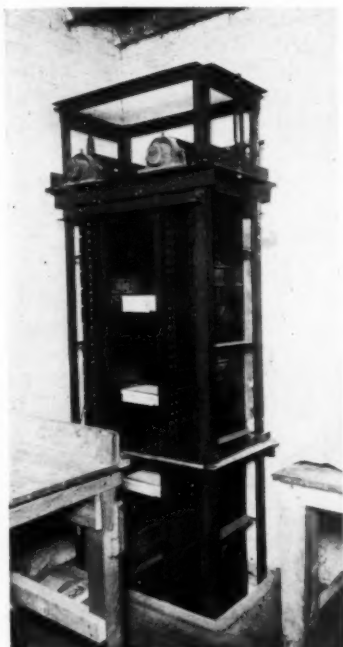
Top of a Subveyor Before the Enclosing Partition is Installed
