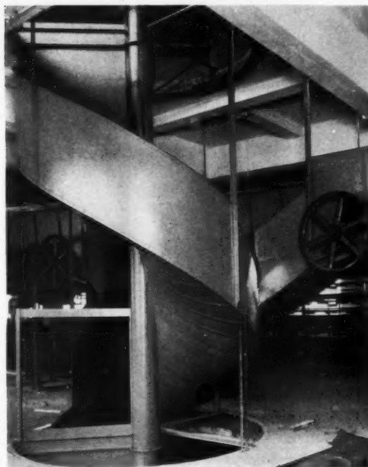
Spiral chutes leading to the wagon space and track floor
