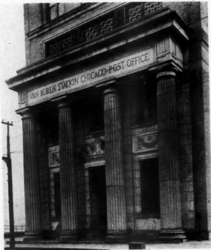
Detail of Entrance, Van Buren Station, Chicago Post Office Graham, Anderson, Probst & White, Architects
