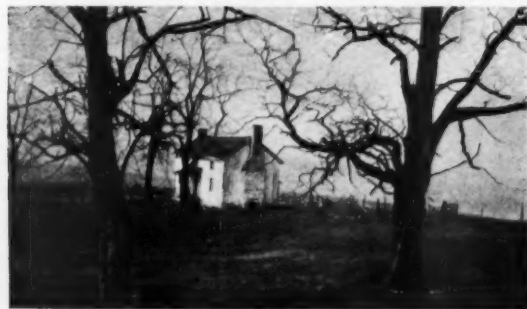
Typical out-building on one of the old plantations
