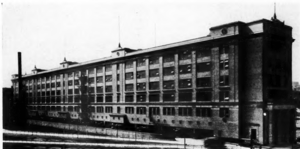
Van Buren Station, Chicago Post Office Graham, Anderson, Probst & White, Architects
