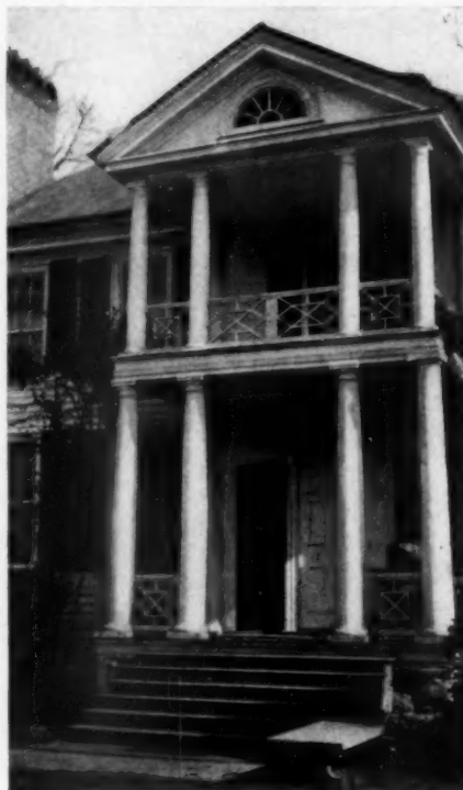
Detail of Entrance, "Tallwood"
