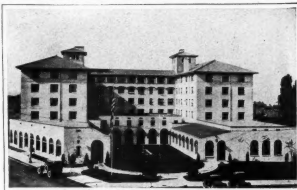
LEWIS-CLARK HOTEL, Lewiston, Idaho: Kirtland Cutter, Spokane, Architect; Hucker & Co., Spokane, Jobbers; Jas. Smythe Plumbing & Heating Co., Spokane, Plumbers; Hurley-Mason, Spokane, Contractors
