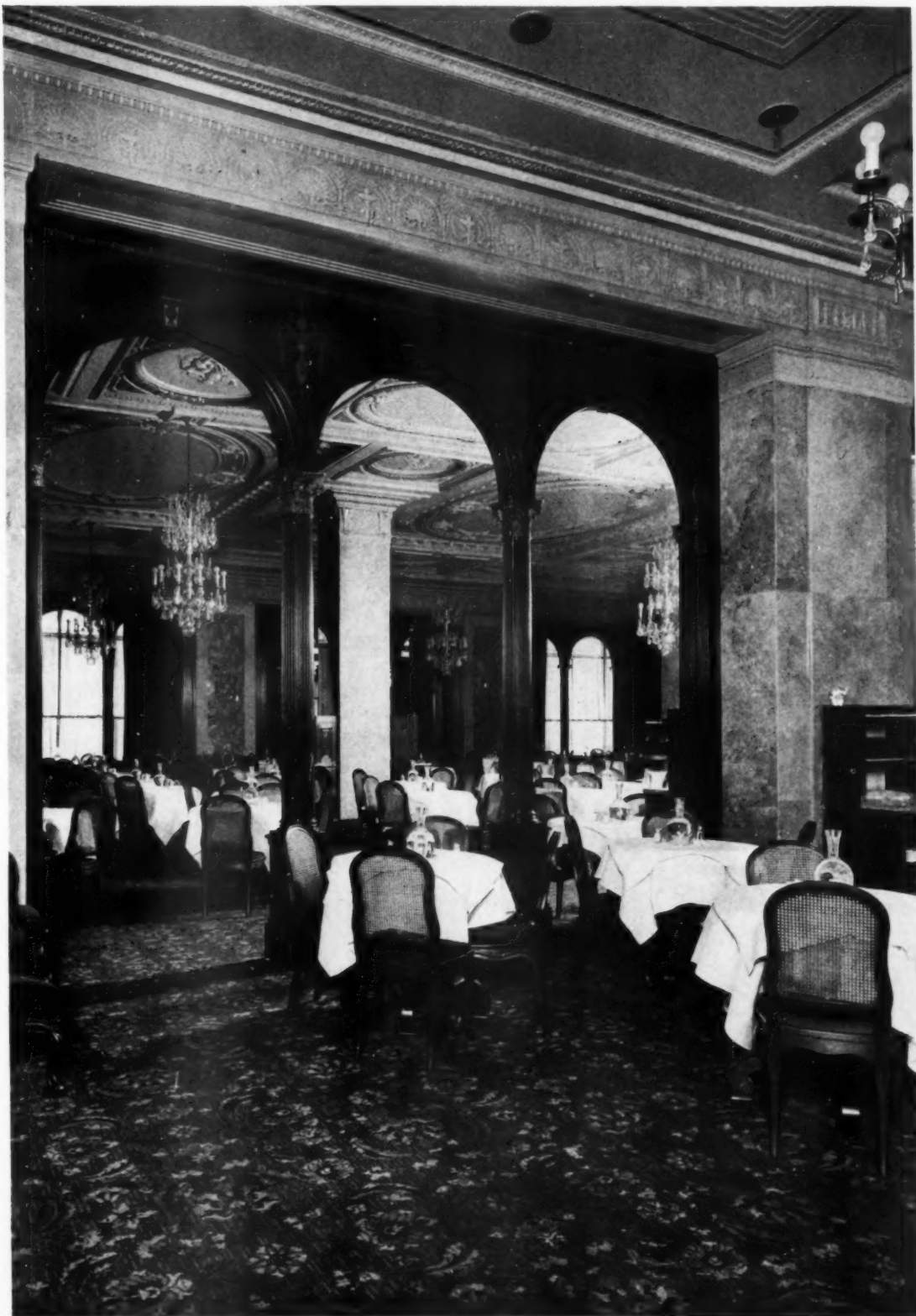
MAILLARD'S RESTAURANT, MADISON AVENUE, NEW YORK BUCHMAN & KAHN, ARCHITECTS
