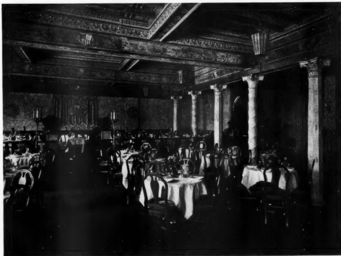
MAILLARD'S RESTAURANT, MADISON AVENUE, NEW YORK BUCHMAN & KAHN, ARCHITECTS
