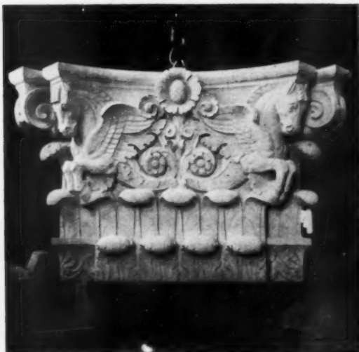
Fig. 4. Corinthian Cap, carved from a single block of limestone
