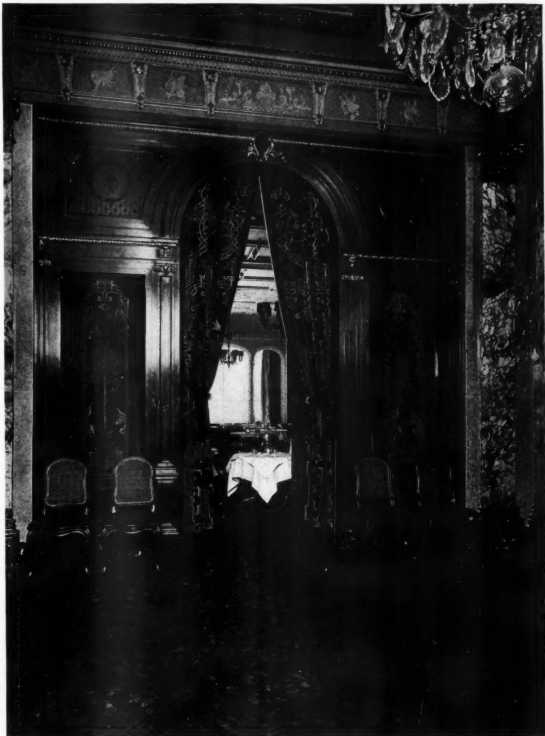
MAILLARD'S RESTAURANT, MADISON AVENUE, NEW YORK BUCHMAN & KAHN, ARCHITECTS
