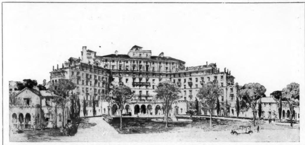
WESTCHESTER BILTMORE COUNTRY CLUB, Rye, New York; Warren & Wetmore, Architects E. Smolka Plumbing Supply Co., Jobbers; Jarcho Bros., Plumbers
