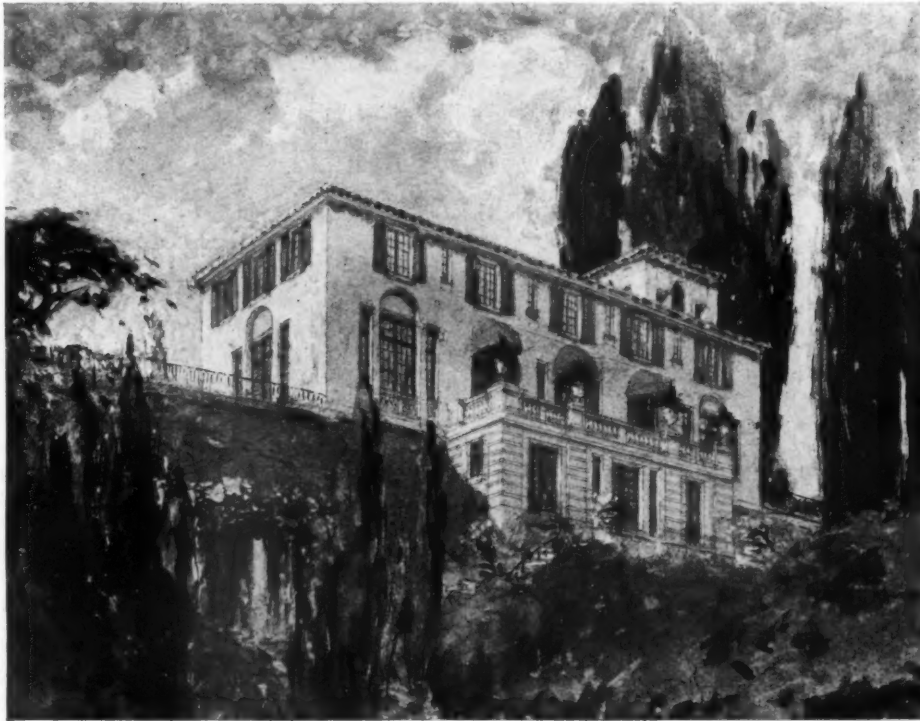
A house at Ann Arbor, Mich. Childs & Smith, Architects
