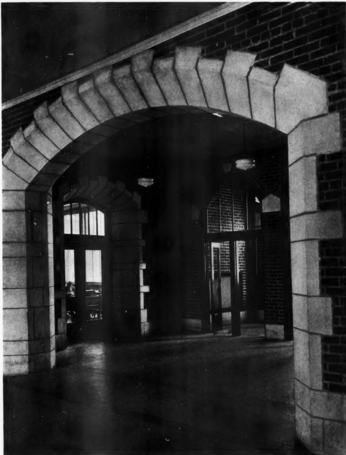
VESTIBULE AND LOBBY UNDER TOWER SENIOR HIGH SCHOOL, BAY CITY, MICH. PERKINS, FELLOWS & HAMILTON, ARCHITECTS
