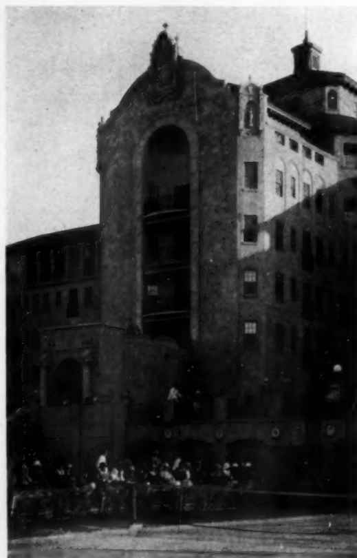
Central Detail. Tennis Courts in foreground
