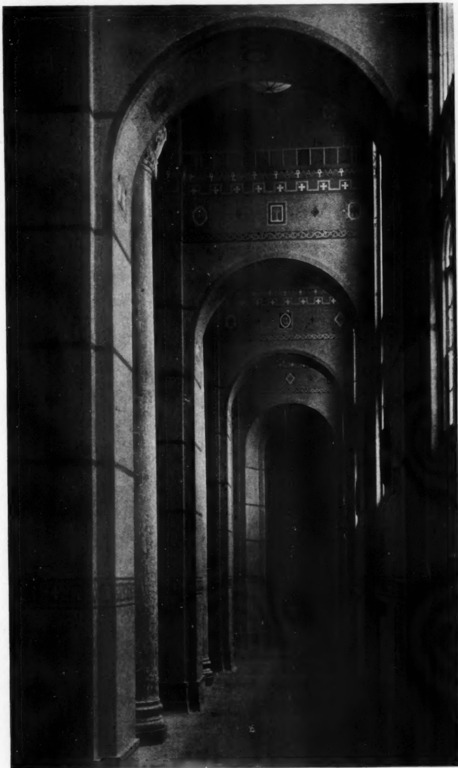
One of the side aisles of the nave. The walls were built on the line of the buttresses and not the piers. The buttresses were pierced and this space used for an aisle leaving the floor of the church proper free for pews
