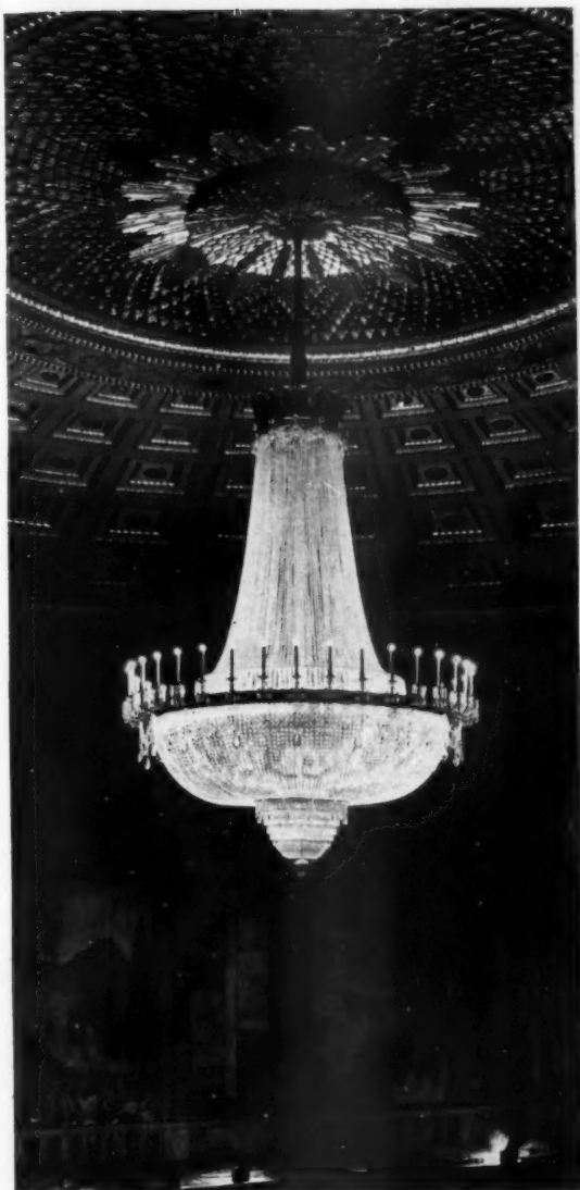
The great chandelier which is the main source of illumination for the Eastman Theatre auditorium. This fixture is about 13 ft. in diameter and 18 ft. high. The low lights have a capacity of about 5 K.W., the high lights of about 15 K.W. and the direct lights of about 8 K. W.
