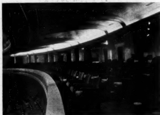
Cove lighting of the mezzanine in the theatre
