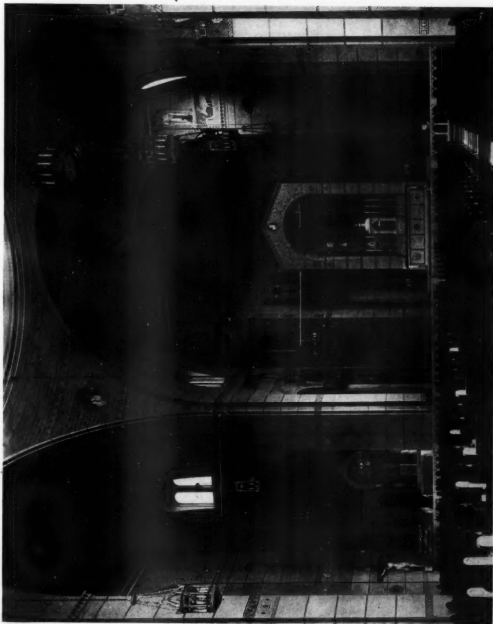
General view of the chancel, the high altar and the chapel of the Blessed Virgin. The altars are marble; the baldachin, walls, arches, cornice of dome and all decorative details are concrete; the ceilings are Guastavino tile
