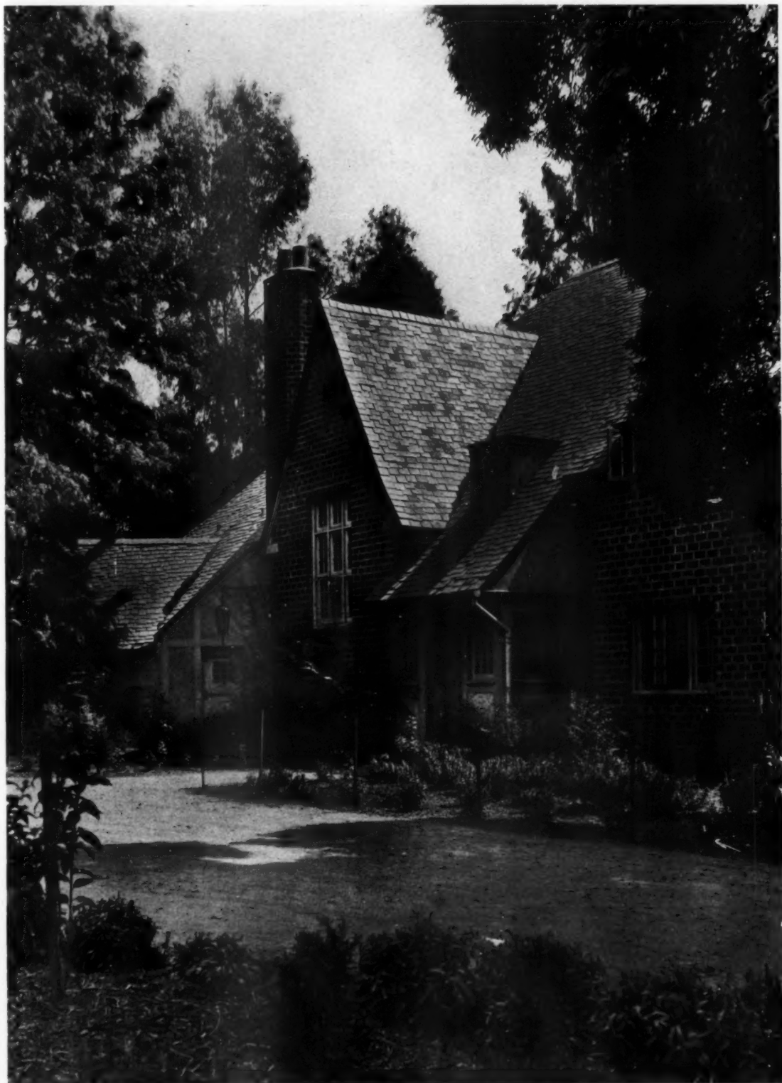
SUPERINTENDENT'S HOUSE, STATE SCHOOL, WHITTIER, CALIFORNIA
