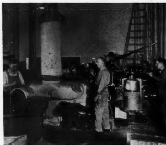
Stereotype casters on the third floor, which by means of a papier-mâché matrix transform the rigid flat type pages into semi-cylindrical plates for the presses
