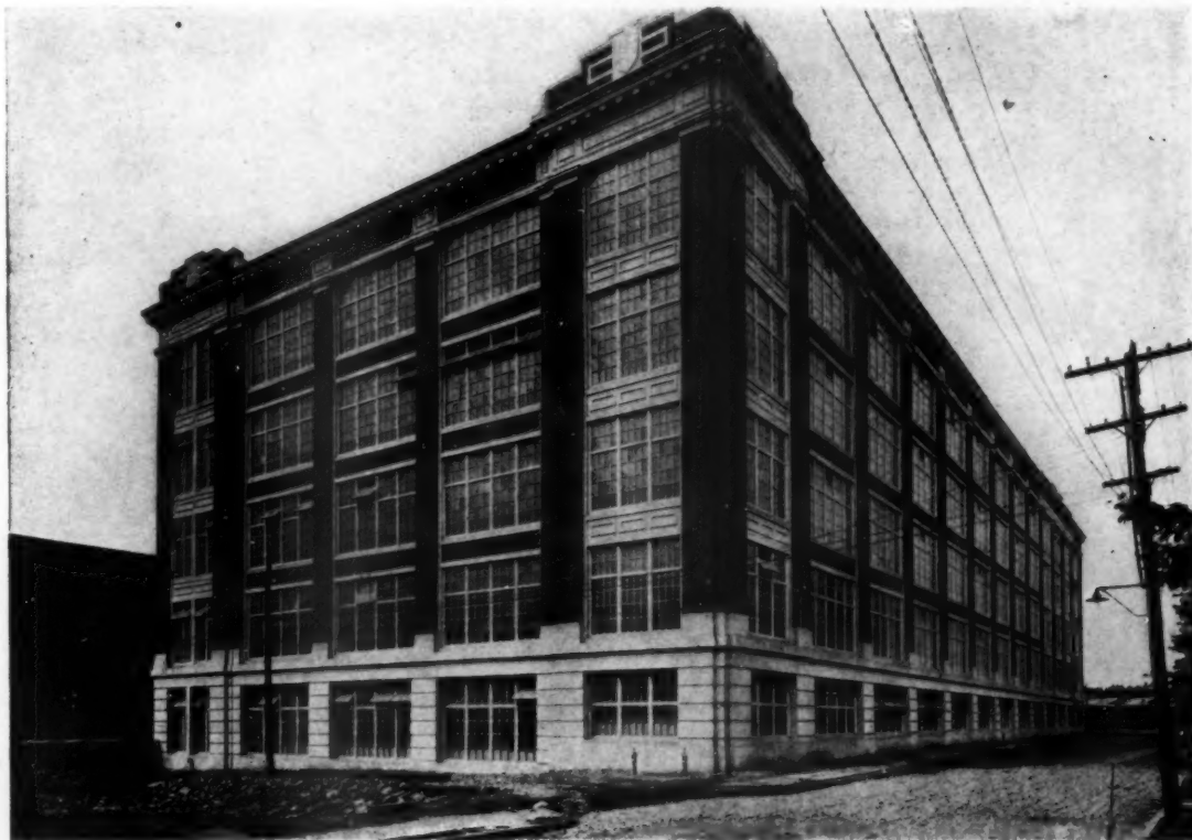
NATIONAL SPUN SILK COMPANY'S BUILDING, NEW BEDFORD, MASS.
