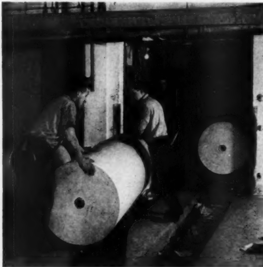
Depressed industrial railway in basement, on which trucks transport rolls of newsprint to the Reel Room on the second floor by means of the elevator
