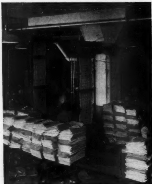
Mailing Room on the first floor, to which the printed and folded papers are delivered by the dispatch conveyors from the Press Room two floors above
