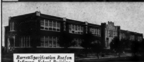
Barrett Specification Roof on Jefferson School Building. Arch.: Layton, Smith & Forsythe. Cont.: C. M. Downing Construction Co. Rfr.: H. A. Turner Sheet Metal Co., all of Oklahoma City.
