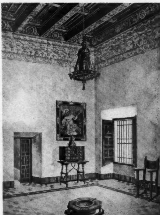
Fig. 1. Salon, Palace of the Duke of Alba, Seville Decorated wooden ceiling, carved plaster frieze, glazed tile floor and base (Courtesy of Wm. Helburn)
