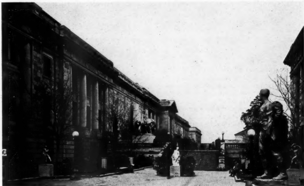
View of Forecourt and approach to the Exhibition
