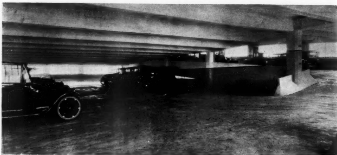
Fort Shelby Garage. Typical Floor looking toward the alley
