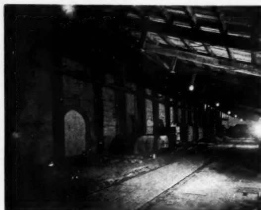
View of a Continuous Kiln, showing chambers closed for burning
