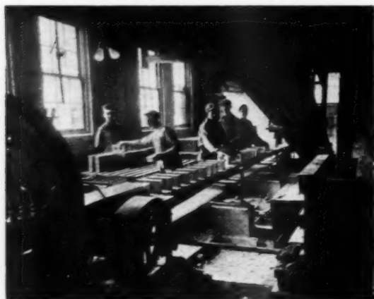
The Brick machine at work, showing the off-bearers
