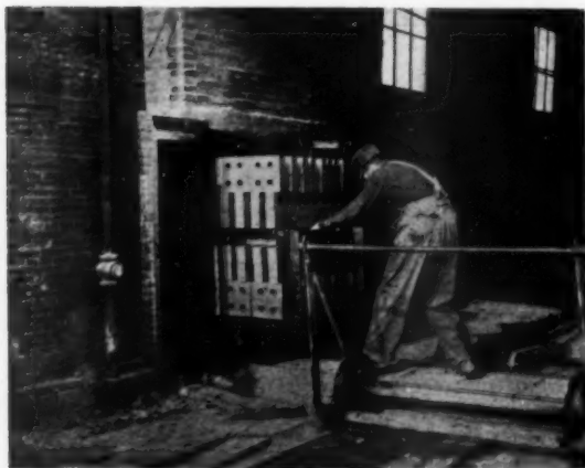
Placing the green brick in the dryer
