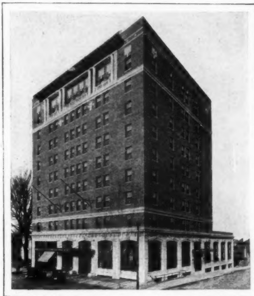
Hotel SHERATON, High Point, N. C., W. L. Stoddard, New York City, Architect; W. G. Cornell Co., Norfolk, Plumber
