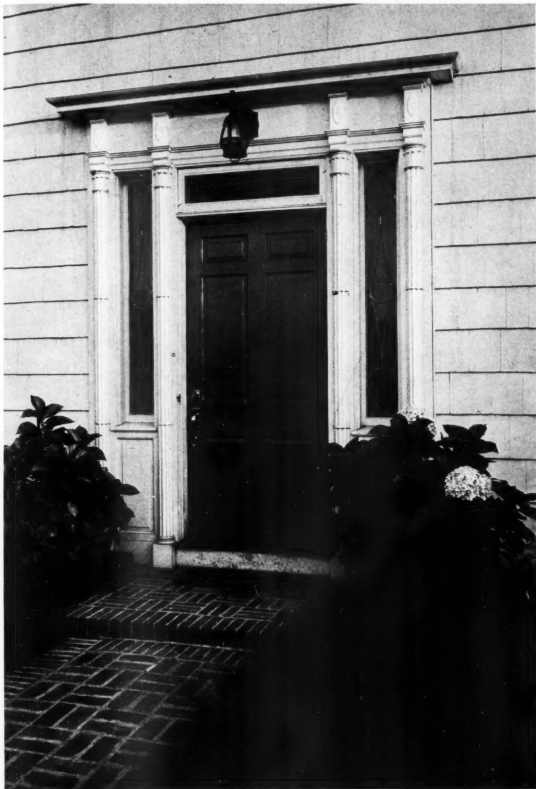
DETAIL OF MAIN ENTRANCE HOUSE OF MALCOLM STEVENSON, ESQ., WESTBURY, L. I., N. Y. DWIGHT JAMES BAUM, ARCHITECT
