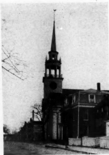
"Old North" Church at Newburyport, Mass. Built 1756
