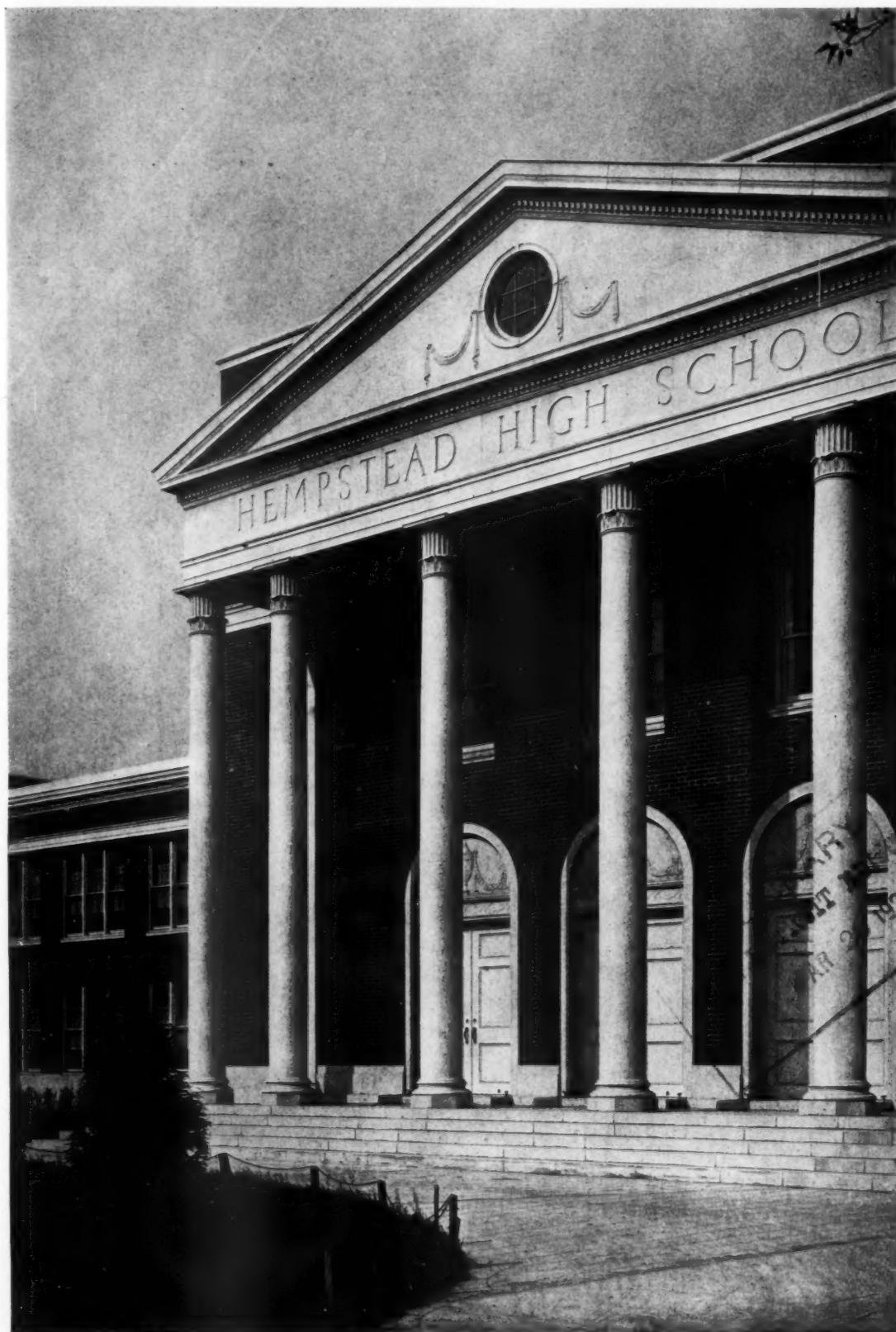
DETAIL OF AUDITORIUM PORTICO
