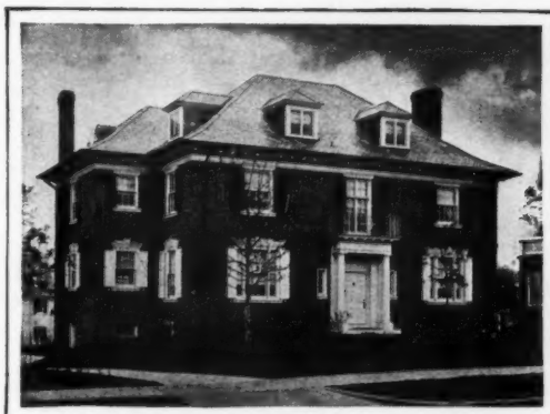
Residence of Walter L. Rathmann, St. Louis: Klipstein & Rathmann, Architects; N. O. Nelson Mfg. Co., Jobber; Ryfel & Rats, Plumber
