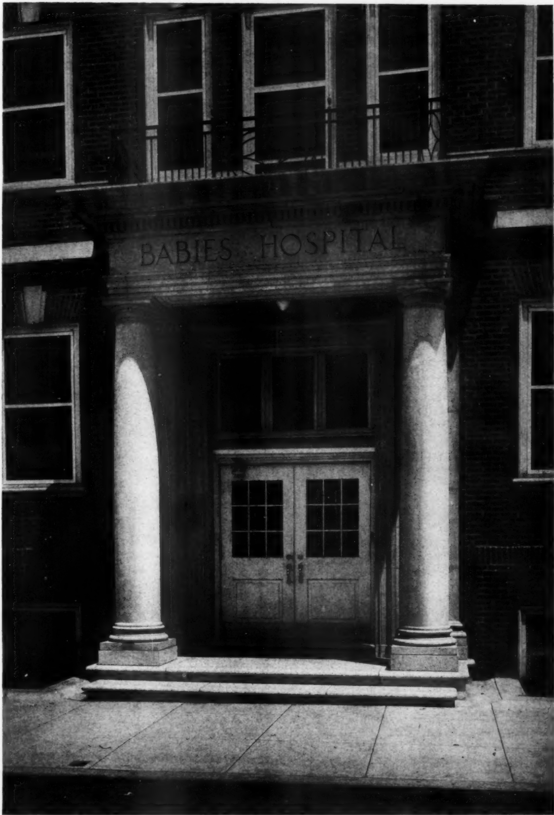
Detail of Main Entrance Babies' Hospital, Philadelphia, Pa. Carl A. Ziegler, Architect
