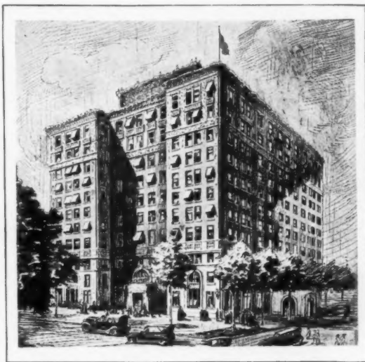
The EMBASSY, Chicago: Walter W. Ahlslager, Architect; Weil-McLain Company, Jobber; Peter K. Clayton, Plumber
