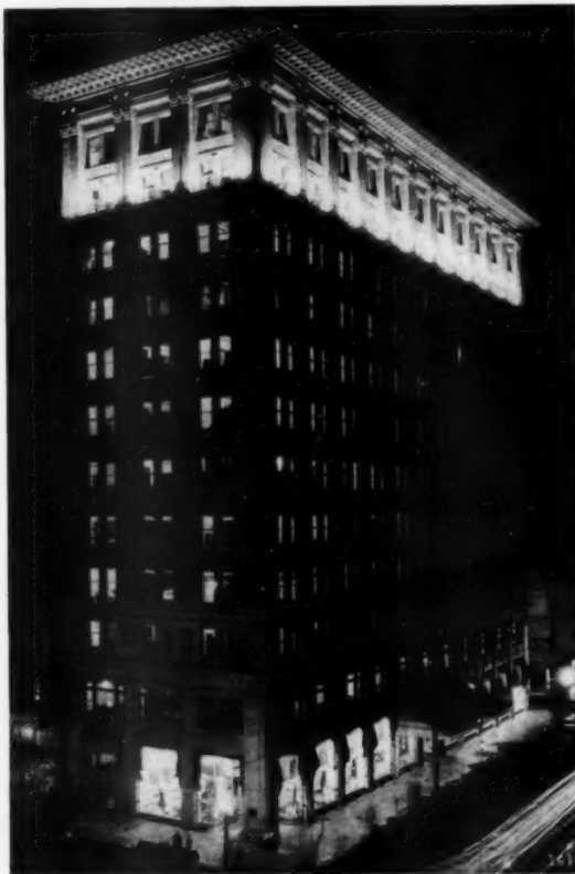
An interesting example of flood lighting
