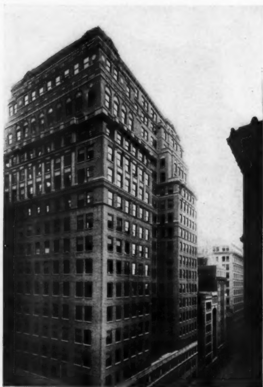
Canadian Pacific Building Starrett & Van Vleck, Architects
