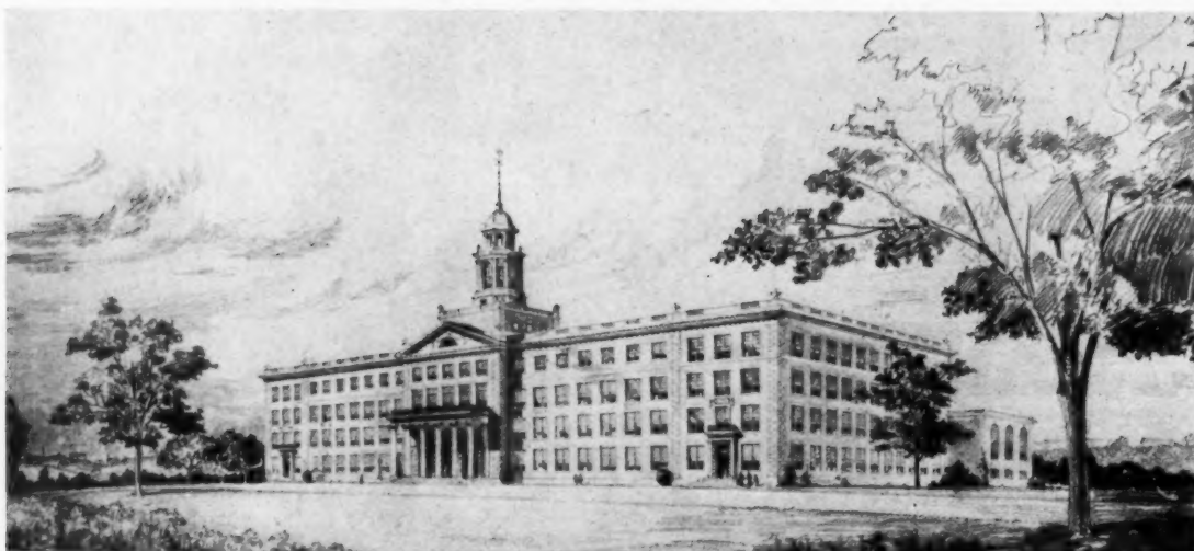
George Washington High School, New York City C. B. J. Snyder, Architect
