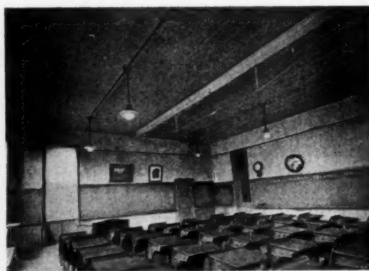
Fig. 8. Outhwaite School, day view of typical test installation, six-unit layout, enamelled and crystal glass enclosing direct lighting globes
