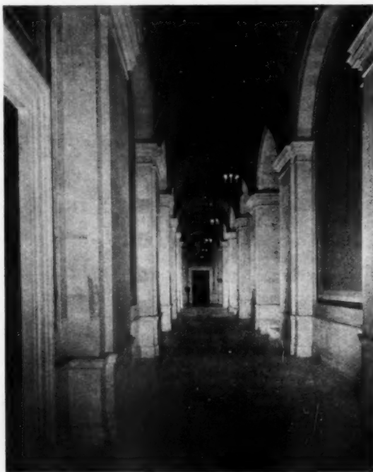
Perspective of Corridor Ceiling, Detroit Public Library, Detroit, Mich.
