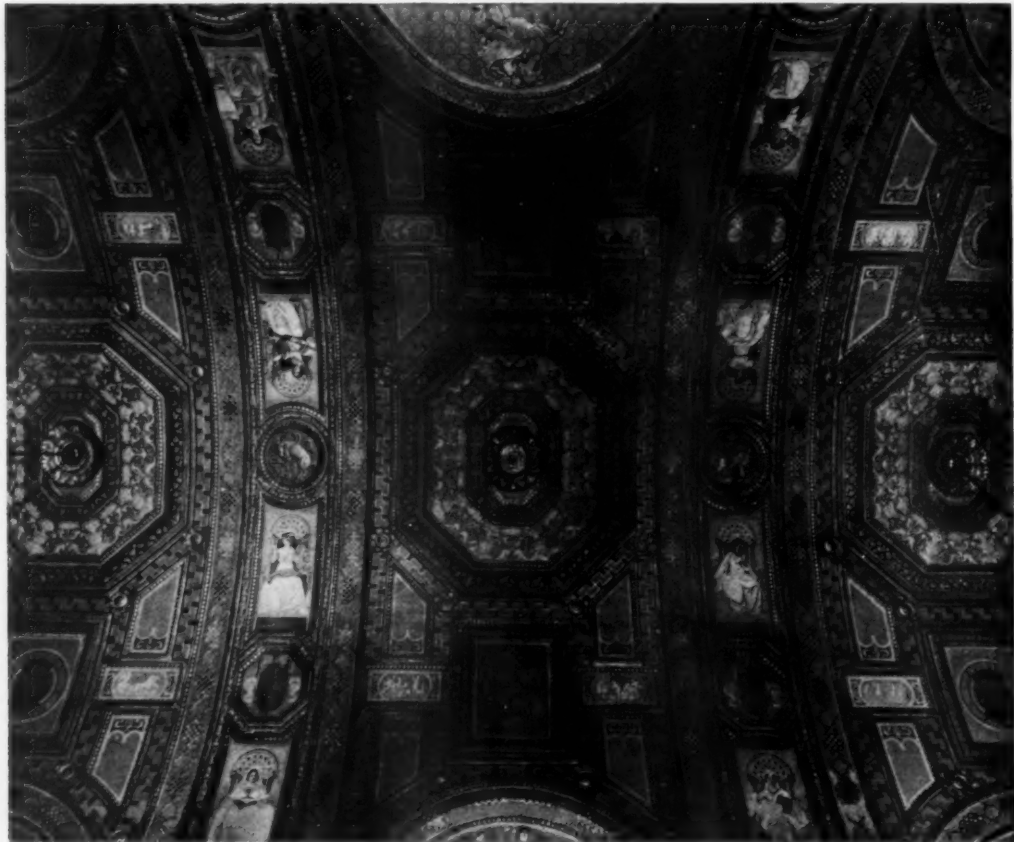
Central Arch of Barrel Vault with detail of ornamentation, Detroit Public Library, Detroit, Mich.
