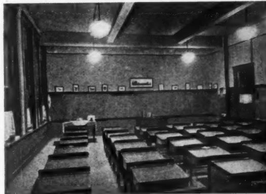
Fig. 9. Murray Hill School, Cleveland, night view of typical class room 33x22 feet, lighted by six 150-watt Mazda C lamps in squat-shape opalescent glass enclosing globes, 16-inch diameter (Trojan)
