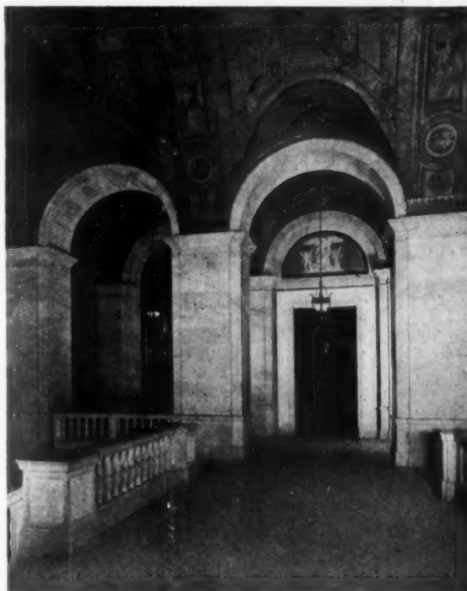
Lateral Section of Barrel Vault showing interlace and inserts, Detroit Public Library, Detroit, Mich.
