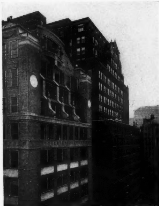
At left: Bar Building Severance & Van Alen, Architects
