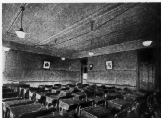
Fig. 7. Outhwaite School, day view of typical test installation, six-unit layout, aquat-shape, opalescent glass enclosing globes
