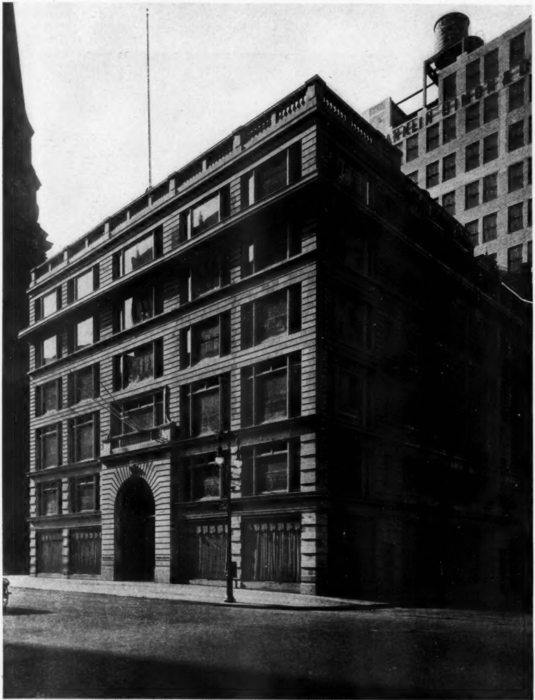
FRANKLIN, SIMON & CO. BUILDING, 414-20 FIFTH AVENUE, NEW YORK NECARSULMER & LEHLBACH, ARCHITECTS AWARDED THE FIRST PRIZE OF THE FIFTH AVENUE ASSOCIATION FOR BUILDINGS ALTERED IN 1922
