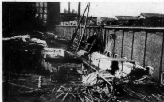
Fig. 5. General view of contractors' plant
