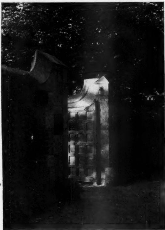
A service gateway to express its character can afford to be somewhat forbidding, and that which would be impossible in a main entrance is here very pleasing
