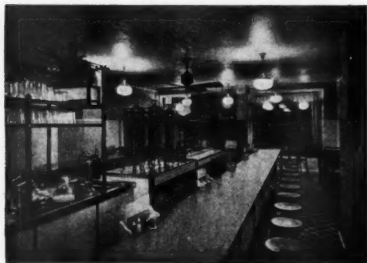
Fig. 2. Interior typical of the commercial restaurant. The low-ceilinged room, in which the luminous type of indirect fixture is suspended on short chains, gives excellent lighting results
