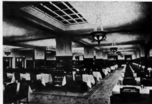
Fig. 7. Restaurant in which the general illumination from luminous indirect fixtures is supplemented by decorative table lamps
