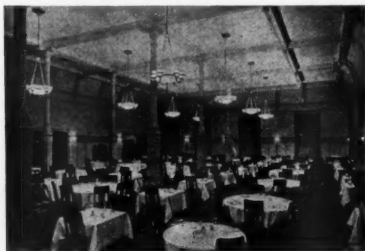
Fig. 8. Principal dining room of the Union League Club, Chicago. An installation illustrating flexibility in the lighting system
