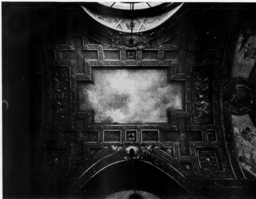
Figs. 6A. and 6B. Detail of ceiling in Grand Foyer, The Century (New) Theater, New York Carrere & Hastings, Architects
