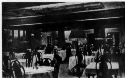
Fig. 10. Good illustration of the use of the indirect portable lamp found in the Stratford Arms Hotel, Milwaukee, Wis.
