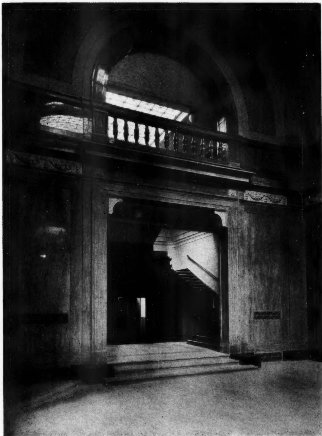
MEMORIAL AUDITORIUM, LOWELL, MASS. BLACKALL, CLAPP & WHITTEMORE, ARCHITECTS
