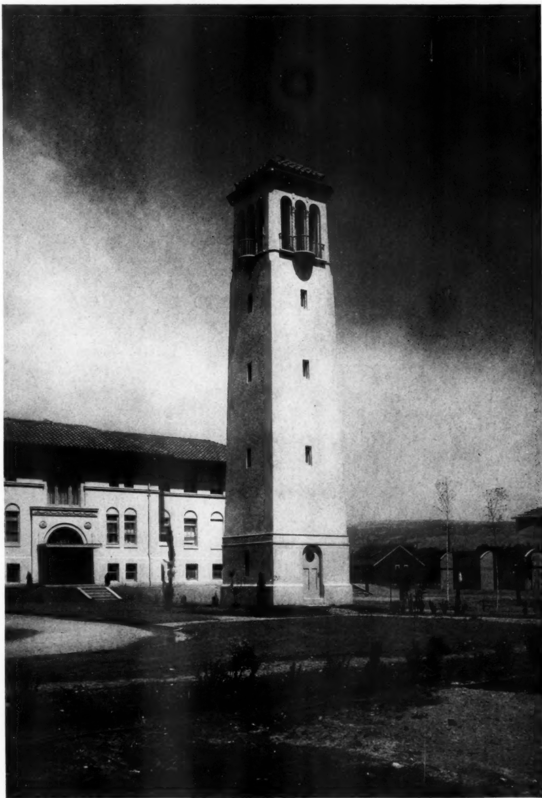
ODD FELLOWS CHILDREN'S HOME, GILROY, CAL. W. H. WEEKS, ARCHITECT
