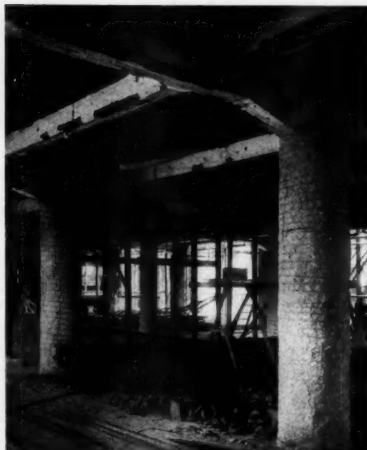
Fig. 4. Columns after damaged concrete was removed in order to make repairs
