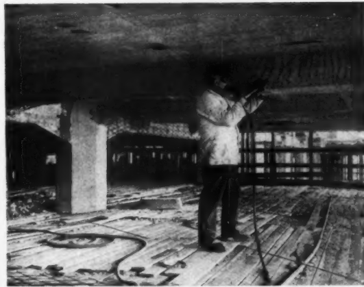
Fig. 6. Using a compressed air chisel to remove damaged concrete. Beams in center ready for Gunite
