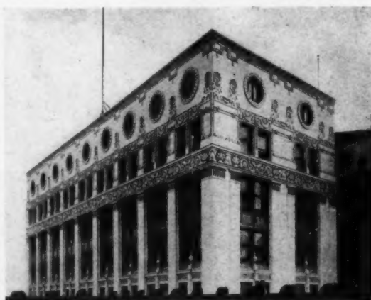
Upper stories of No. 80 Maiden Lane, New York City D. H. Burnham & Company, Architects (View taken from roof of an opposite building)
