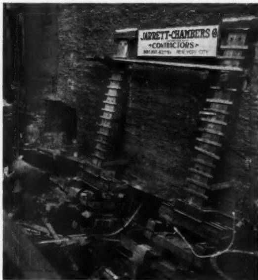
Fig. 7. Spur shores on South wall of old Standard Oil Building, No. 26 Broadway
