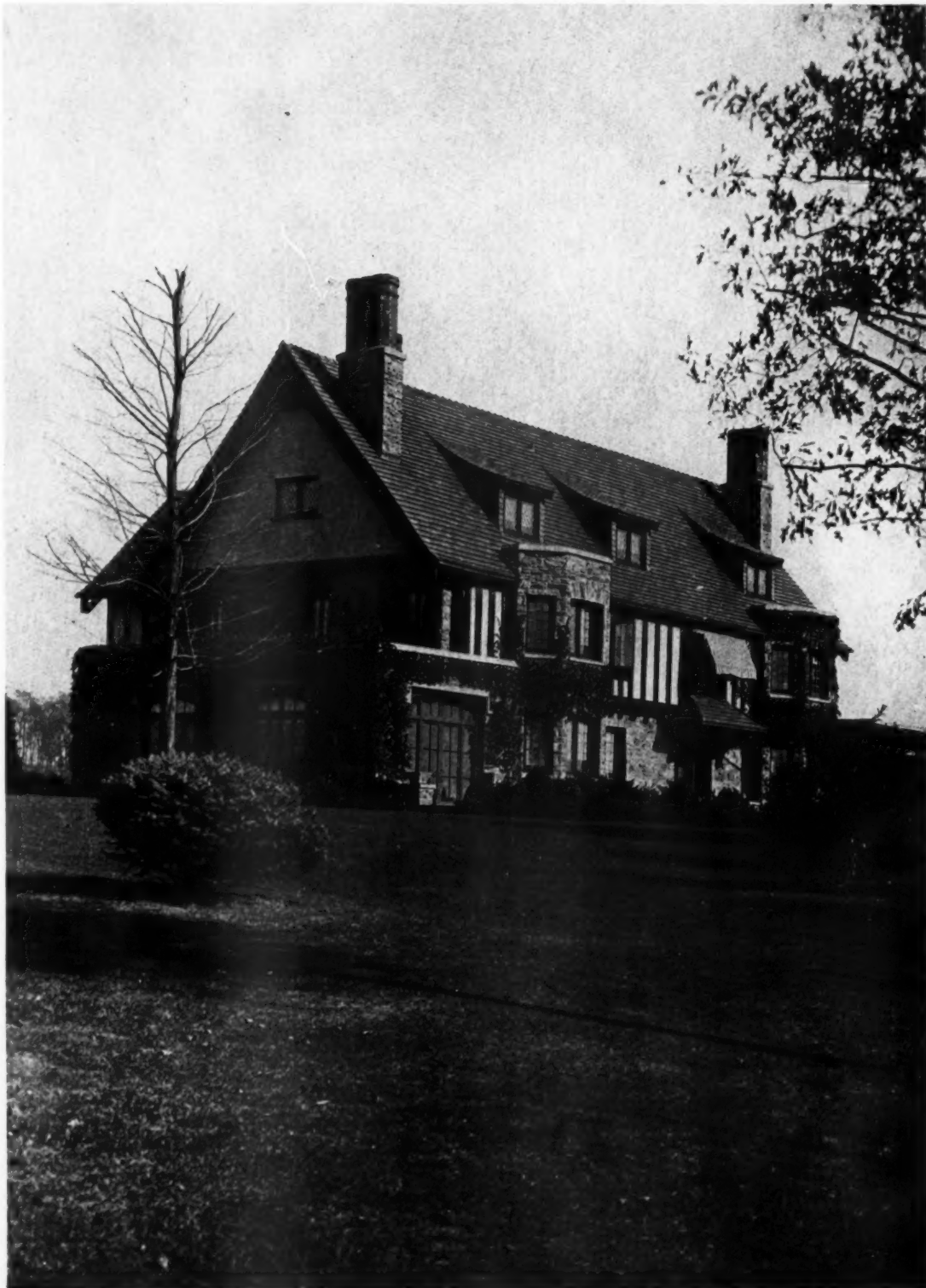
HOUSE IN ABINGTON, PA.
