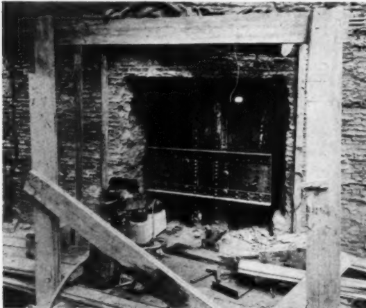
Fig. 14. Method of attaching bracket shore to Column H in south wall of old Standard Oil Building
