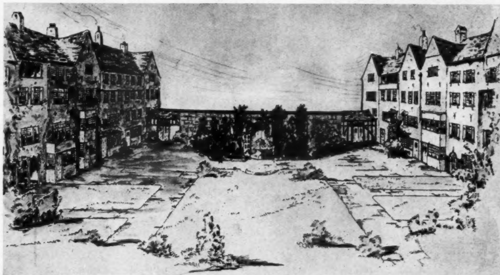
View of interior Court of remodeled block
