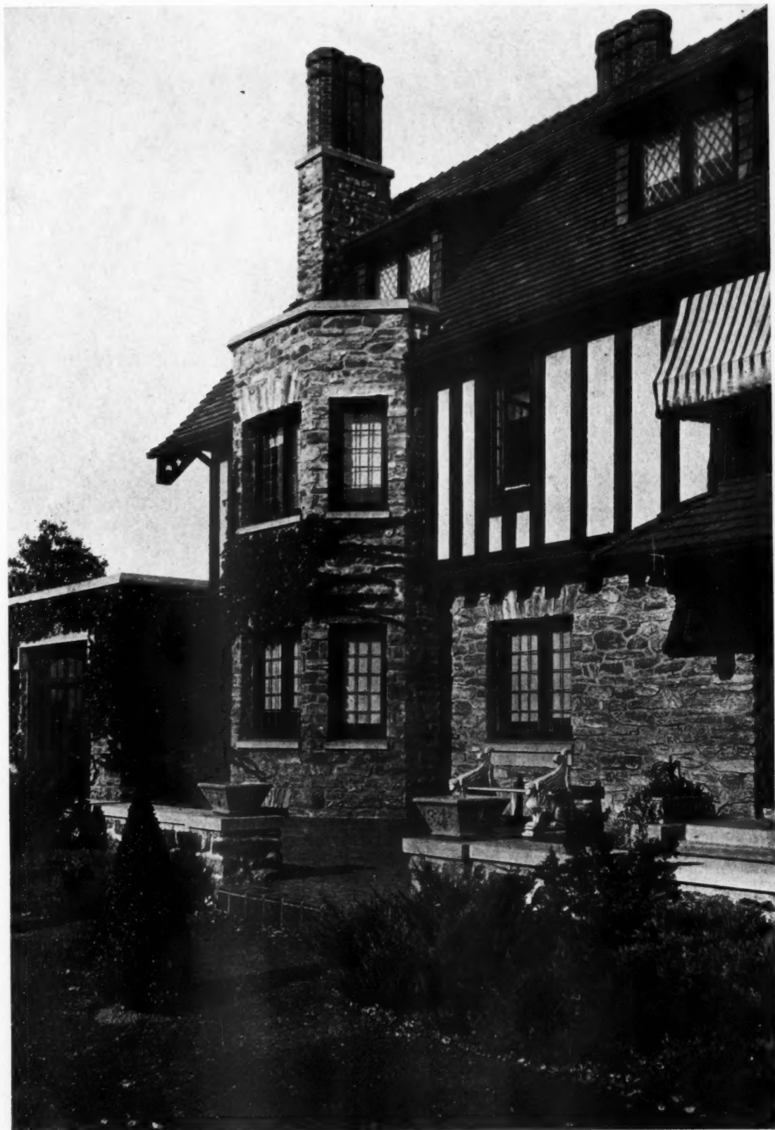
DETAIL OF HOUSE IN ABINGTON, PA.
