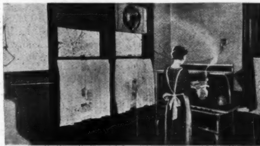
A fan in the kitchen of the home is a necessity and not a mere luxury
