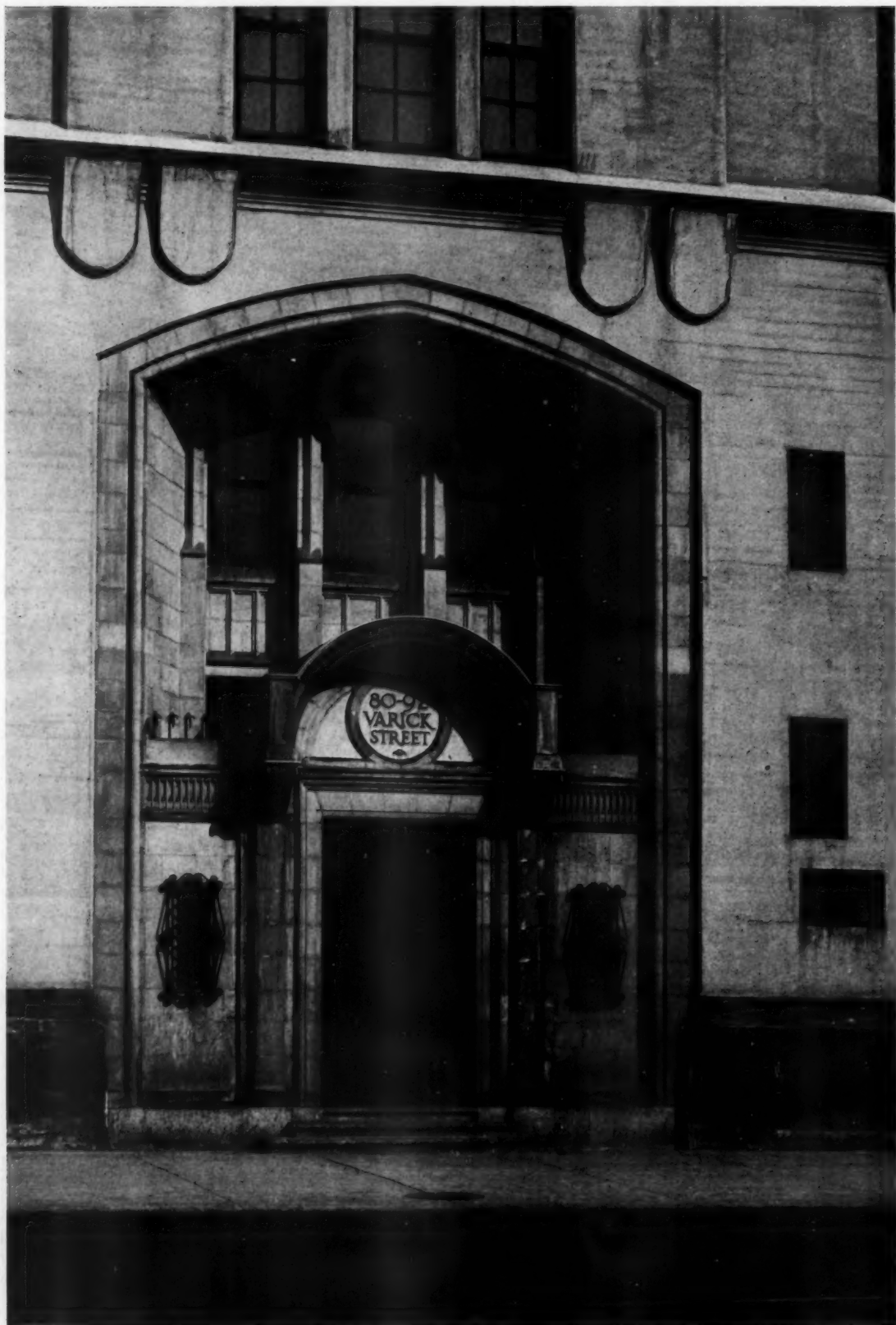
DETAIL OF PRINCIPAL ENTRANCE VARICK STREET BUILDING, NEW YORK HELMLE & CORBETT, ARCHITECTS
