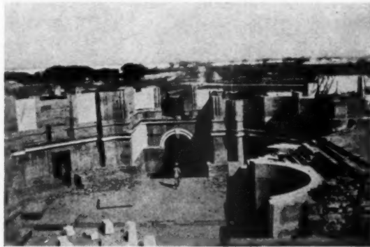
Secretariats, New Delhi Large entrance hall to North block
