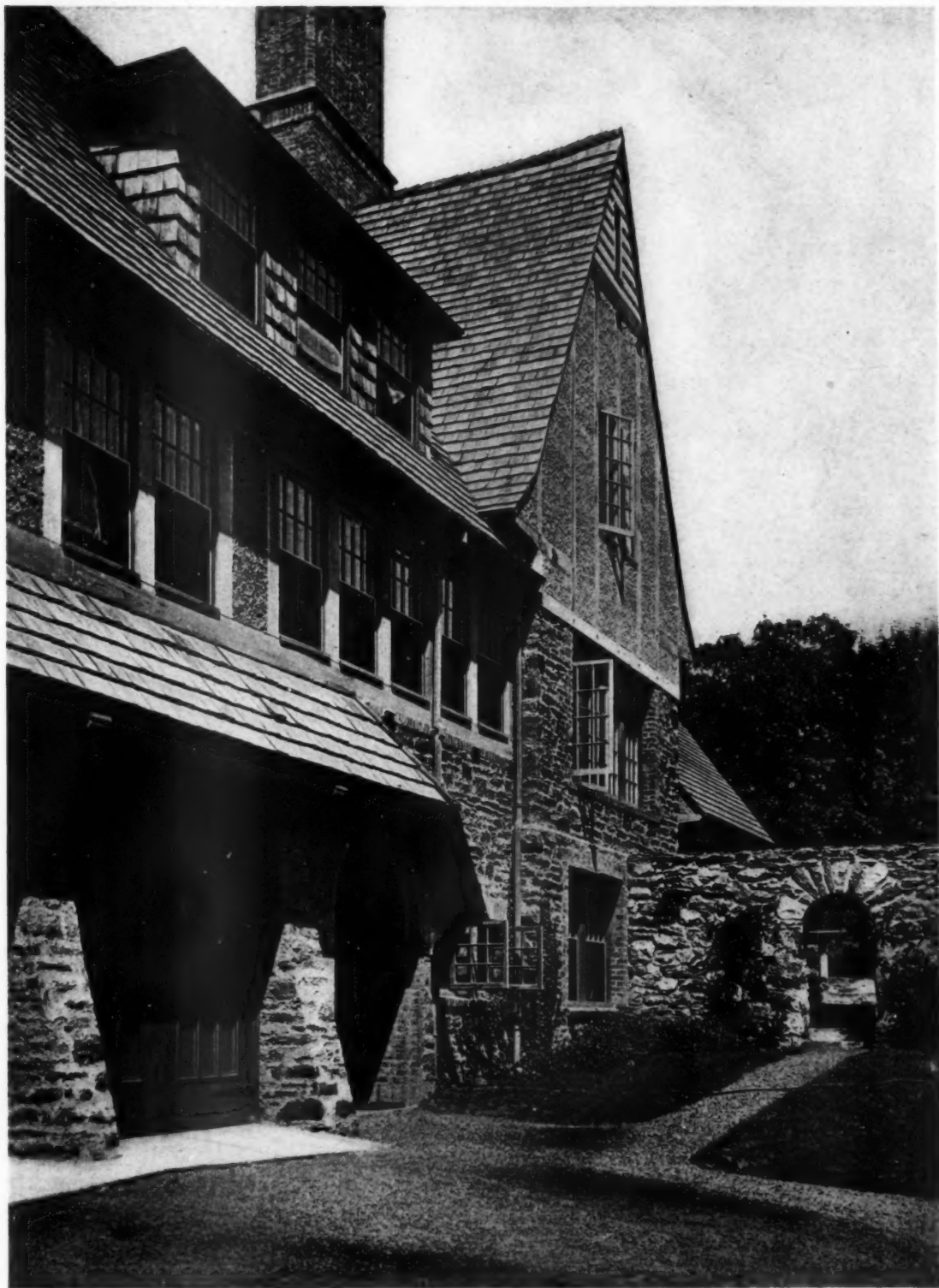
SERVICE ENTRANCE AND GARAGE HOUSE OF LORENZO D. ARMSTRONG, ESQ., RIVERSIDE, CONN. DONN BARBER, ARCHITECT
