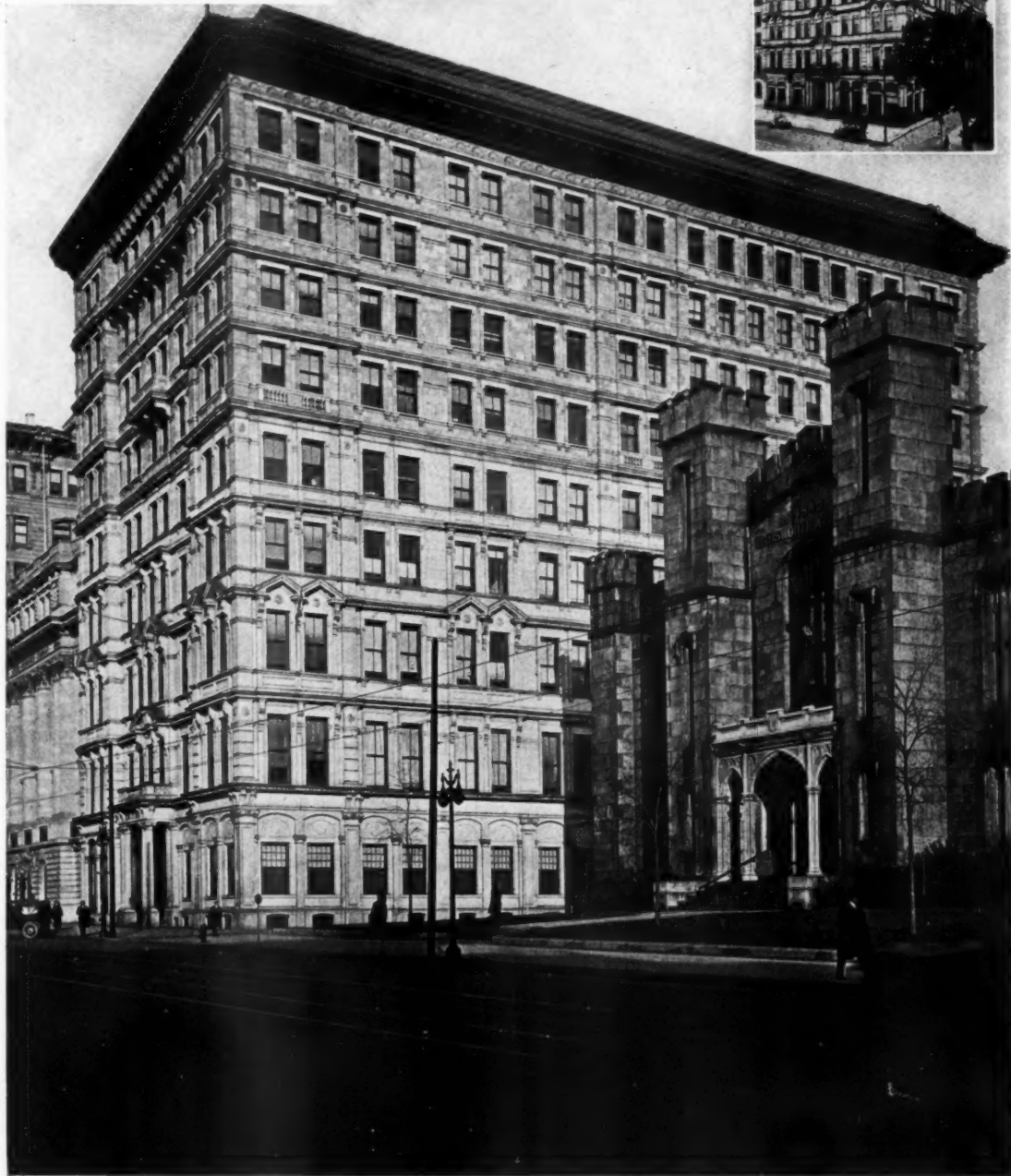
OFFICE BUILDING OF AETNA LIFE INSURANCE COMPANY, HARTFORD, CONN.
