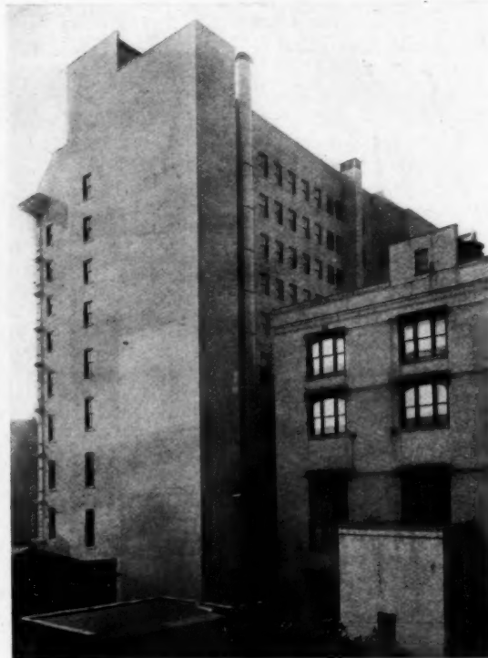
Rear view of completed building of the Aetna Life Insurance Company, Hartford, Conn.
