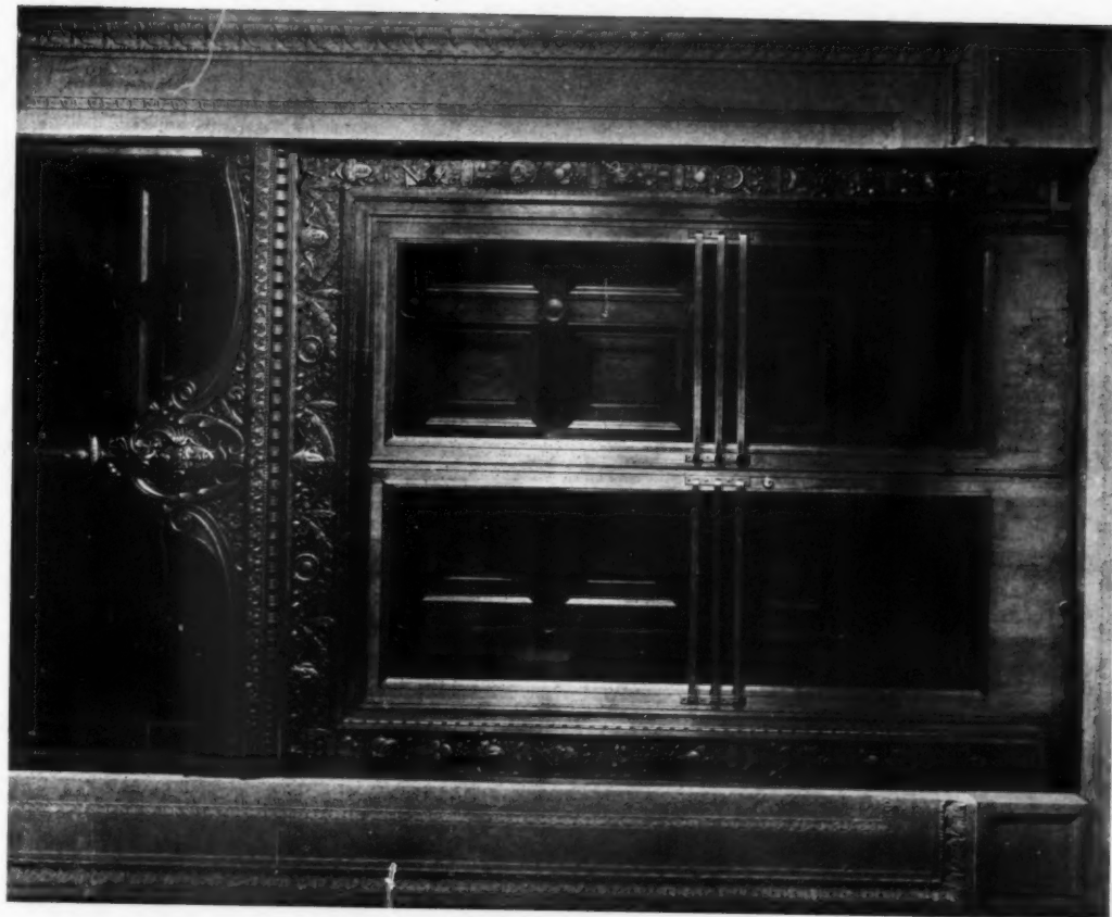
MAIN ENTRANCE DOORWAY TO BANKING ROOM
