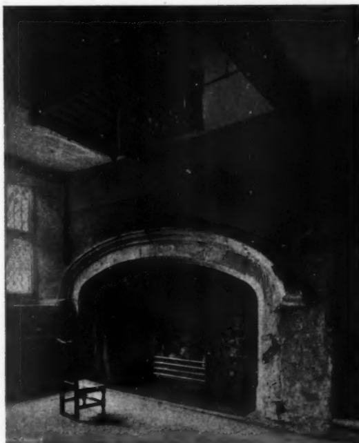
Fireplace in the Kitchen of Plas Mawr, Devonshire, England
