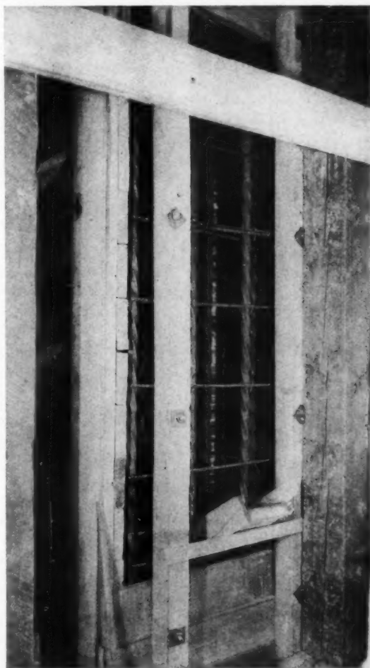
The concrete in the reinforced concrete columns was poured in story-height sections. Aetna Life Insurance Company Building, Hartford, Conn.
