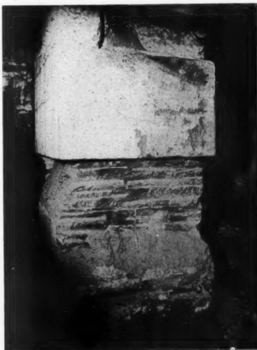
One of the reasons for the adoption of the methods used in adding to the height of the Aetna Life Insurance Building, Hartford, Conn. How many foundations in soft clay would present a similar appearance were they bared for inspection?
