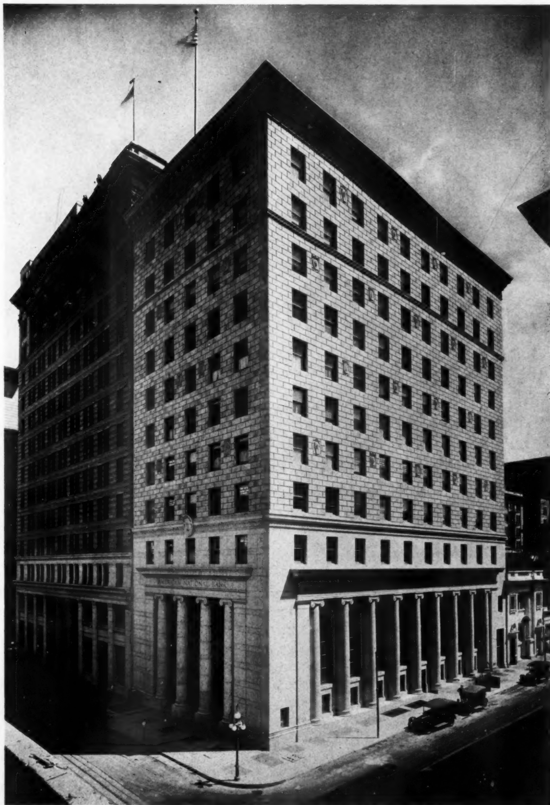
AMERICAN NATIONAL BANK BUILDING, SAN FRANCISCO, CAL. GEORGE W. KELHAM, ARCHITECT
