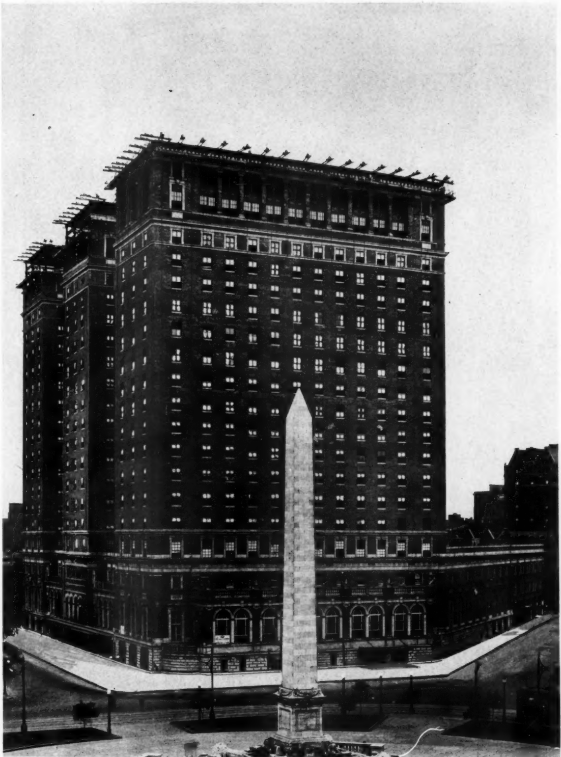
GENERAL VIEW, TAKEN DURING CONSTRUCTION NEW HOTEL STATLER, BUFFALO, N. Y. GEORGE B. POST & SONS, ARCHITECTS
