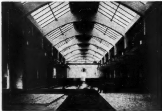
Fig. 22. Interior of warehouse for steel rods in Europe. The arch is a logical form for a roof of concrete
