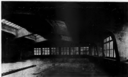
Sixty-five-foot concrete arch span on top floor of Sharman Garage, Salt Lake City, Utah. Miller, Woolley & Evans, Architects
