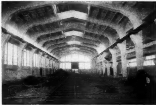
Seventy-foot concrete arch span in foundry of the Garfield Smelting Co., Garfield, Utah
