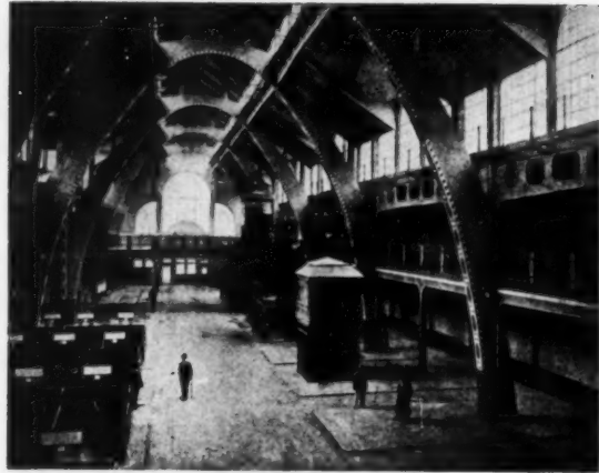
Market Hall, Breslau. A notable example of the adaptability of reinforced concrete as a construction material
