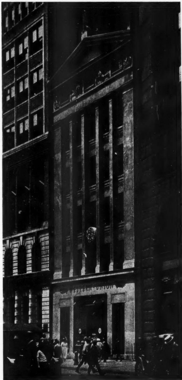
OCEAN CABLE BUILDING OF THE WESTERN UNION TELE- GRAPH CO.
