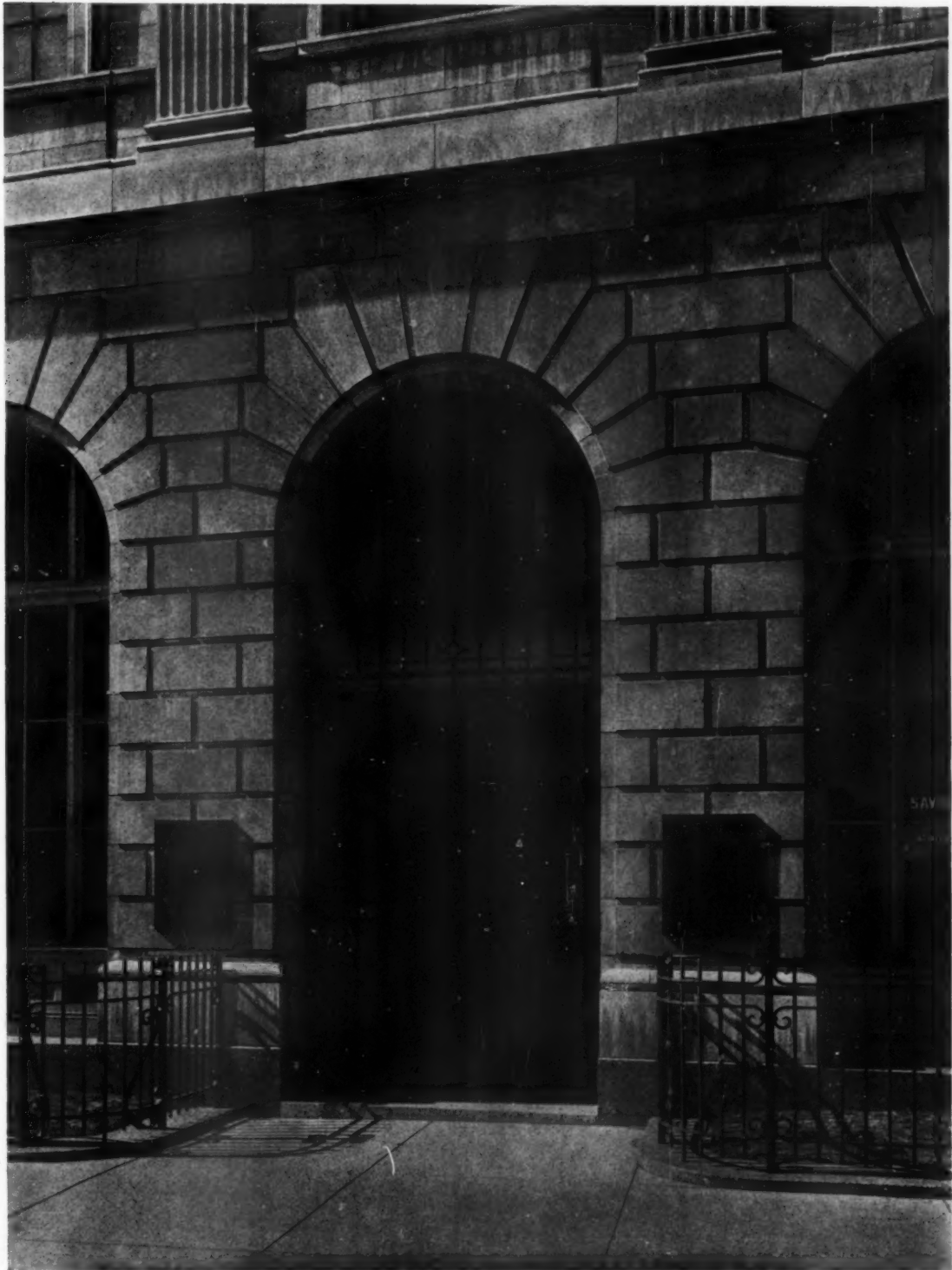
MAIN ENTRANCE WATERBURY NATIONAL BANK, WATERBURY, CONN. CASS GILBERT, ARCHITECT
