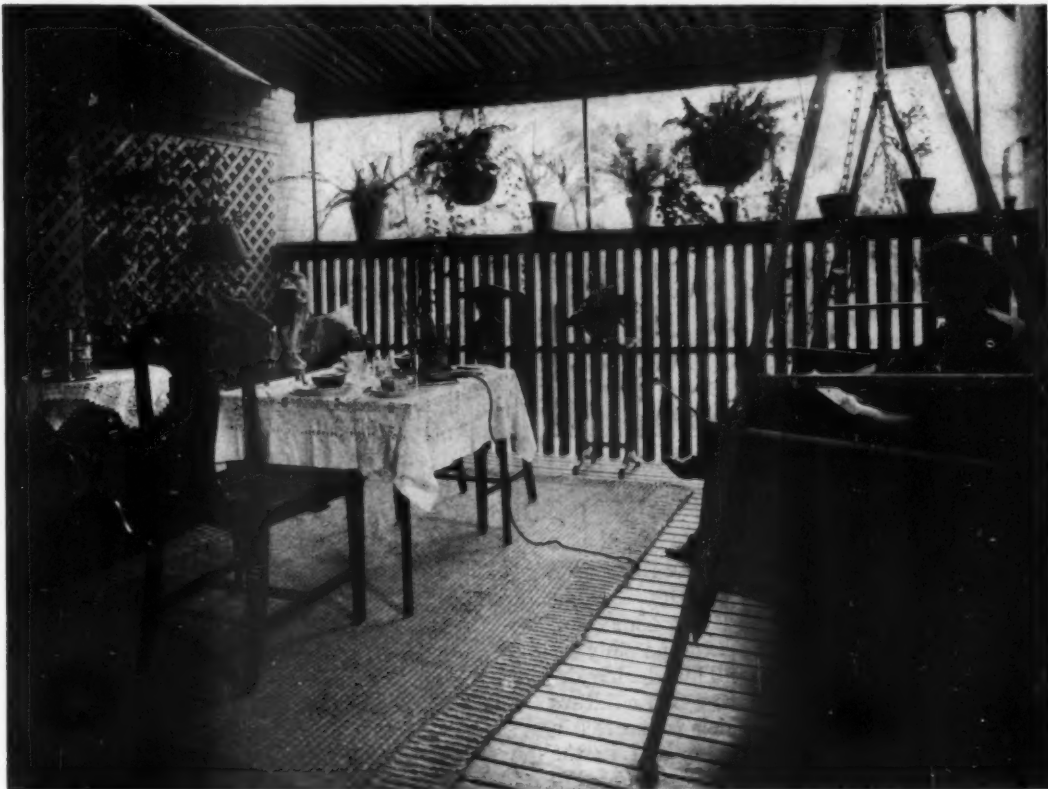
Some wires, some buttons and a switch or two in combination with appropriate furnishings make the home porch a formidable competitor of country vacation resorts. The wire should go through the rug. It is dangerous as shown here
