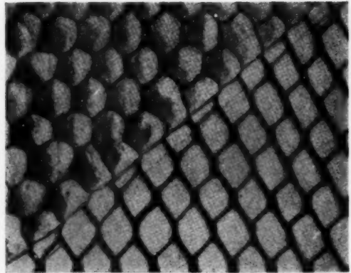
ENLARGED VIEW SHOWING KEYING OF PLASTER ON THE METAL LATH
