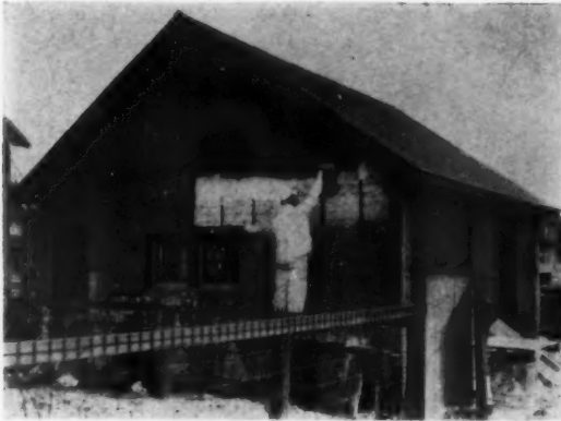
STUCCO GARAGE OF BACK PLASTERED TYPE IN THIS INSTANCE THE BACK PLASTER WAS APPLIED BEFORE THE EXTERIOR COATS
