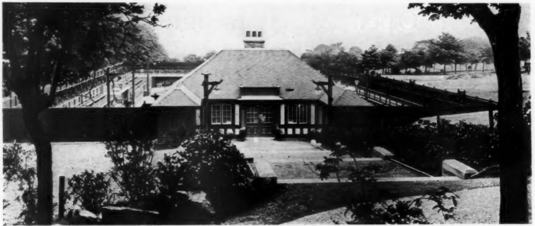
ENTRANCE TO THE POOL. THE BALCONIES ON EITHER SIDE ABOVE THE SWIMMING POOL LEVEL CAN BE SEEN.
