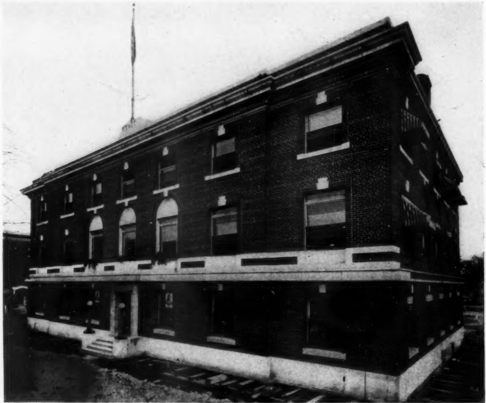
FRONT ELEVATION. THE BUILDING WAS OCCUPIED DURING THE ENTIRE PERIOD OF MOVING.
