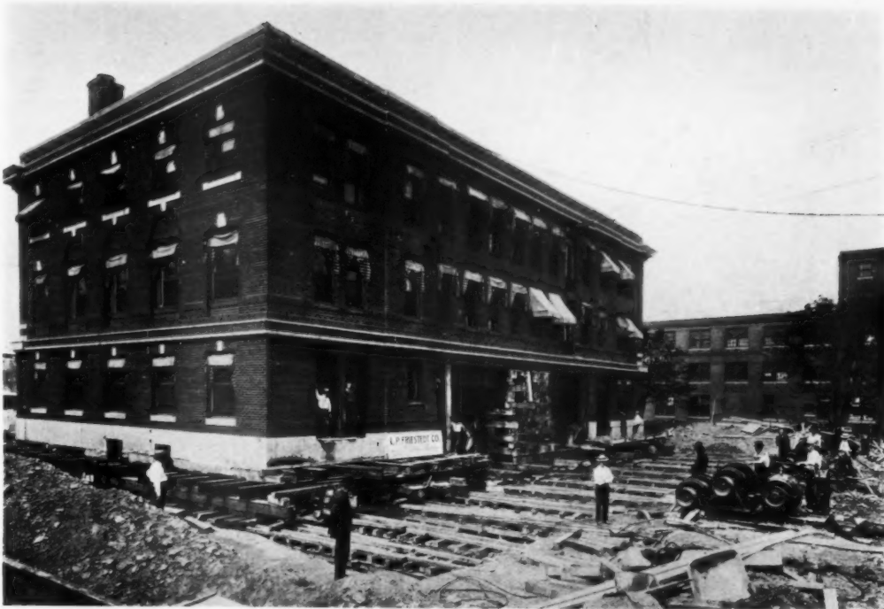
REAR AND SIDE VIEW. ELECTRIC HOISTING ENGINES USED IN SUCCESSFULLY MOVING THE BUILDING, SHOWN TO THE RIGHT.
