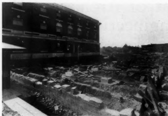
CONDITION ON JULY 23, 1919. THE BUILDING HAS BEEN MOVED SUFFICIENTLY TO CLEAR THE OLD CONCRETE FOUNDATIONS SHOWN IN THE FOREGROUND.
