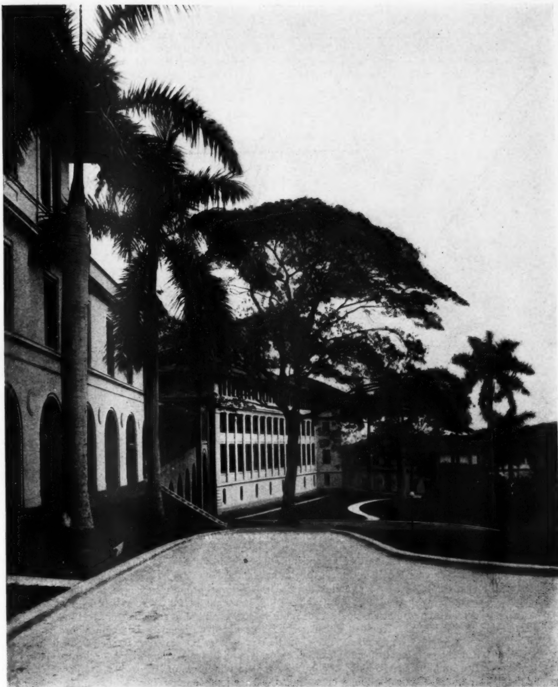
GENERAL VIEW, SHOWING KITCHEN, MESS SECTION C AND LABORATORY ANCON HOSPITAL, ANCON, PANAMA CANAL ZONE SAMUEL M. HITT, ARCHITECT
