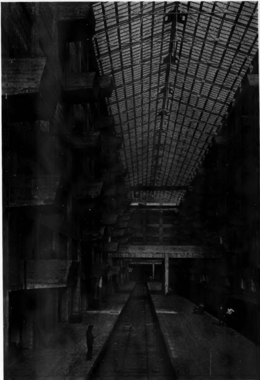
Court in Building B, showing arrangement of cantilever balconies served by travelling cranes, handling supplies direct from rail to warehouse. PLATE 184
