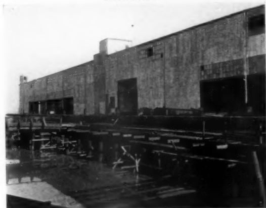
No. 5. NEARING COMPLETION, MAY 28, 1919. PROGRESS PHOTOGRAPHS OF WHARF AND WHARFHOUSE, UNITED STATES ARMY SUPPLY BASE, NEW ORLEANS, LA.
