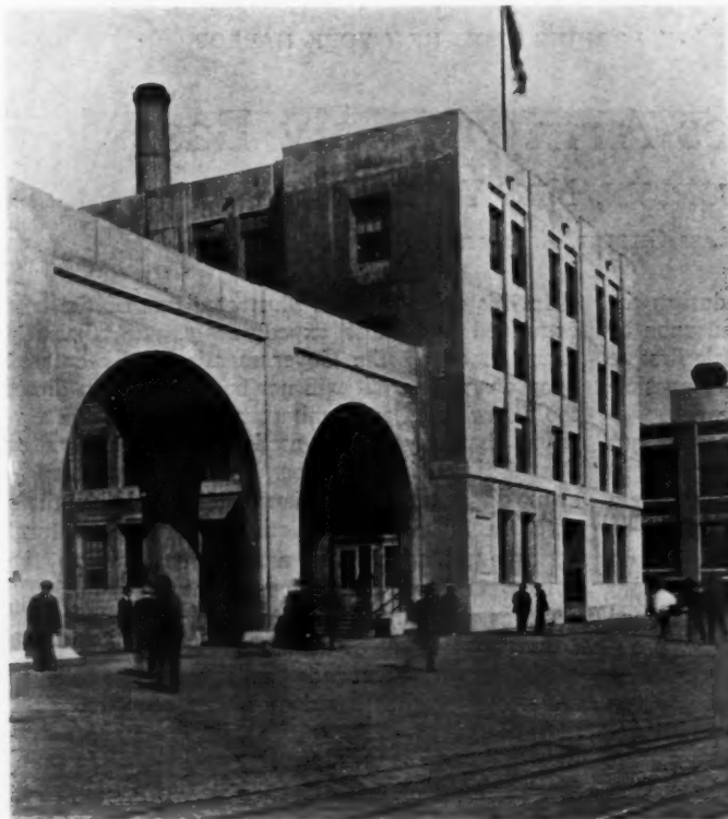
A WAREHOUSE AND CONNECTING BRIDGE
