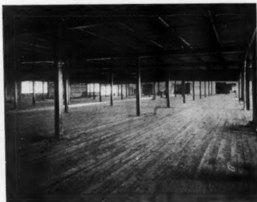
No. 6. INTERIOR VIEW OF COMPLETED WHARFHOUSE.
