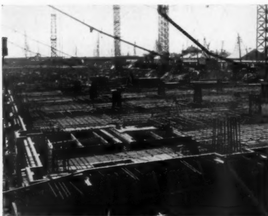
WHARFHOUSE No. 3 AS IT APPEARED JANUARY 15, 1919.
