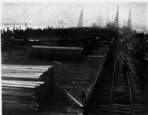
No. 2. FEBRUARY 19, 1919. DECKING LAID OVER COMPLETED PILES.
