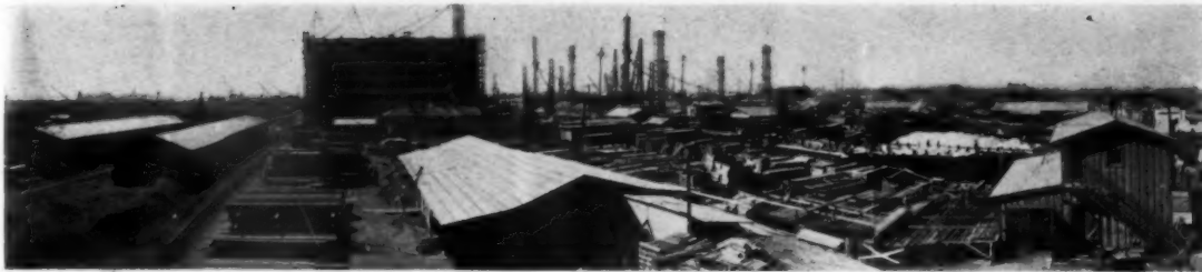
WAREHOUSES 1, 2 AND 3 AS THEY APPEARED JANUARY 15, 1919.
