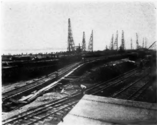
No. 1. JANUARY 22, 1919. PILE DRIVING IN PROGRESS.
