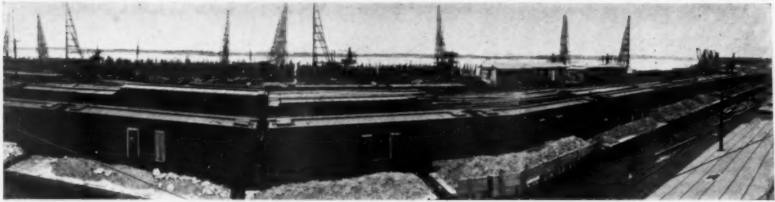
PANORAMIC VIEW LOOKING TOWARD SITE OF WHARFHOUSE, SHOWING CONDITION JANUARY 15, 1919. NOTE THE GREAT NUMBER OF PILES BEING DRIVEN TO SUPPORT THE WHARF AND WHARFHOUSE
