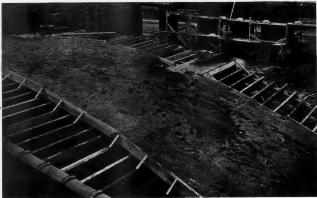
METHOD OF CONDUCTING TEST ON LATTIS ROOF TRUSS, BROOKLYN BUREAU OF BUILDINGS Wet sand, weighing 87 lbs. per cu. ft., used for loading purposes. Total load on truss at completion of test 121 tons.
