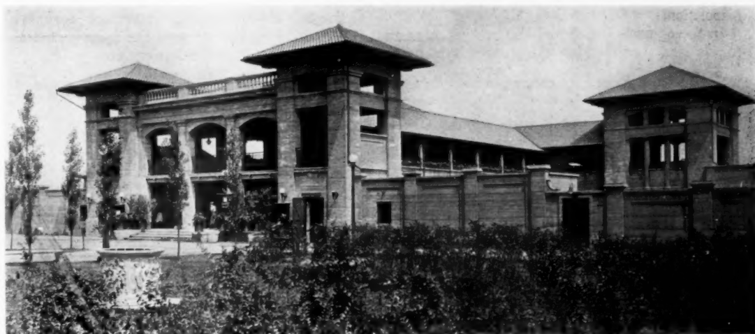
Parkside Entrance, Jackson Park Bathing Pavilion. Planned and constructed under the supervision of the Engineering forces of the South Park Commissioners. Entrance to the dressing rooms and lockers is through the door in first story of the towers. Checkroom windows on either side. Entrance to the store and service rooms and to the upper promenade is through the three center openings. Concrete wall enclosing the men's and women's sections at left and right of center pavilion.
