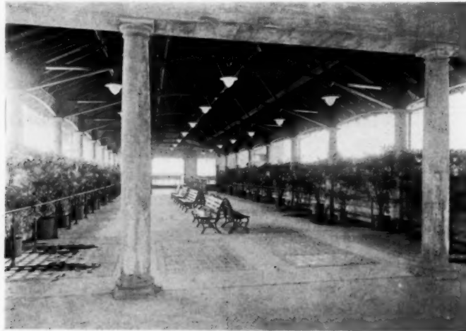
Covered promenade over the service and store rooms. Men's section at the right and women's section at the left behind and below the concrete parapet walls. View looking toward the parkside entrance.
