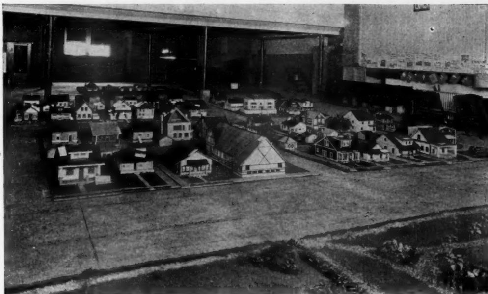
VIEW SHOWING WELL CONSIDERED GROUPING OF TYPES
