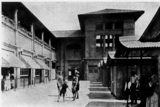
View in women's section looking toward the only exit to the beach. Dressing rooms and lockers at the right; service and store rooms to the left. Persons on upper promenade prevented from observing this section by the concrete parapet walls.
