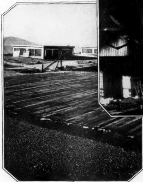
Exterior view of new piers built largely of Redwood
