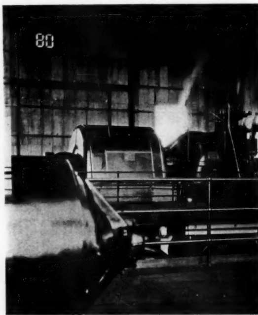
Portion of turbine room, looking north; 10,000 K.W. turbine is to the rear. Temporary north wall construction shown in background.
