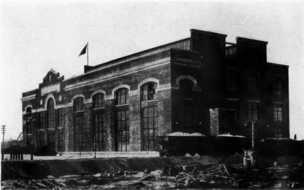
The Erie Lighting Company's Plant just after completion. DAY & ZIMMERMANN, INC., ARCHITECTS AND ENGINEERS
