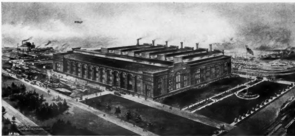
POWER PLANT—ERIE LIGHTING CO., ERIE, PA. DAY & ZIMMERMANN, INC., ARCHITECTS AND ENGINEERS
