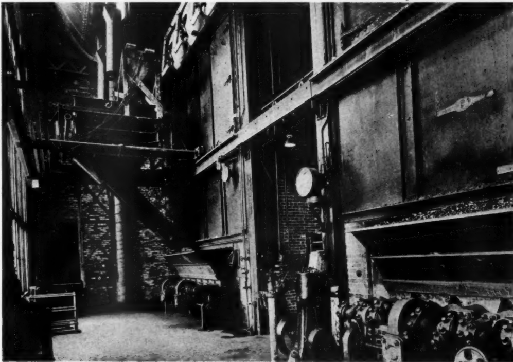
A corner of the boiler room, showing overhead coal bunkers, coal chutes, weighing carry; stoker hoppers and underfeed stokers.
