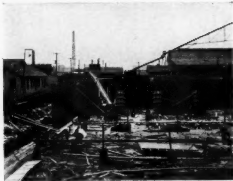
No. 2. Early days of construction.
