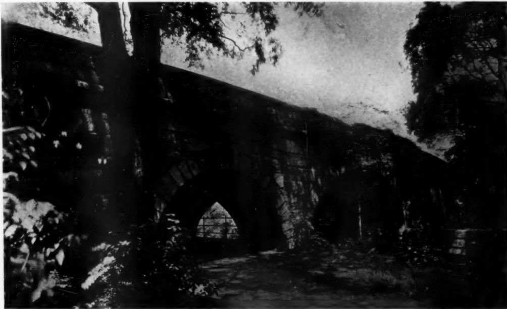
BRIDLE PATH BRIDGE
