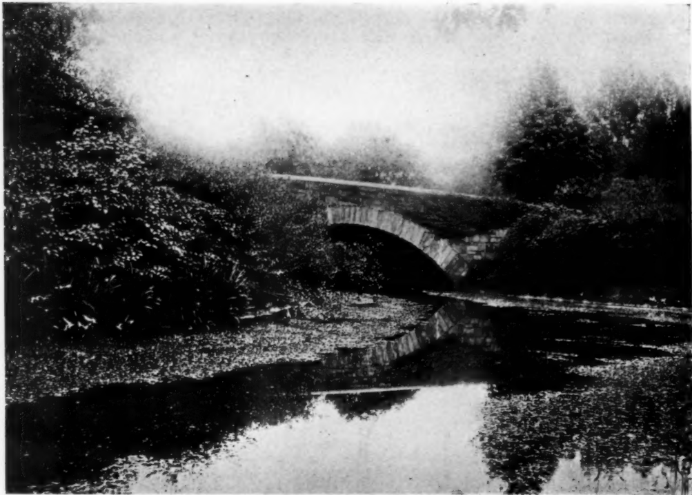
BELLEVUE STREET BRIDGE
