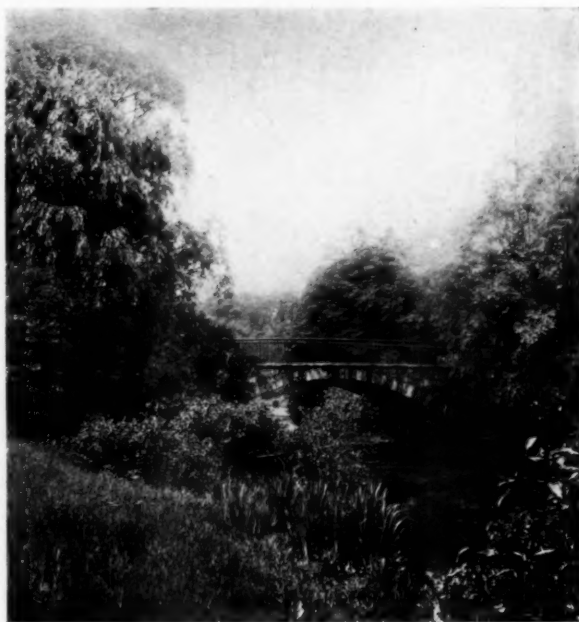
BERNIER STREET FOOT BRIDGE
