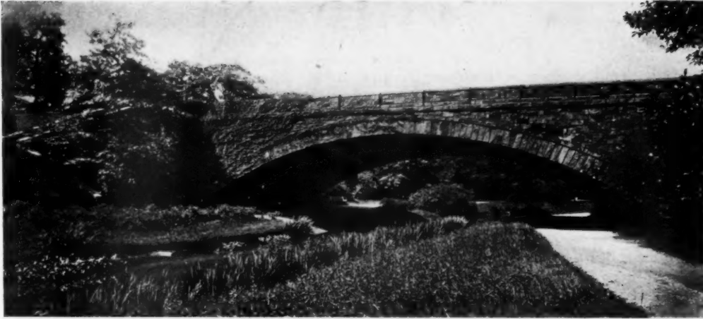
LONGWOOD AVENUE BRIDGE
