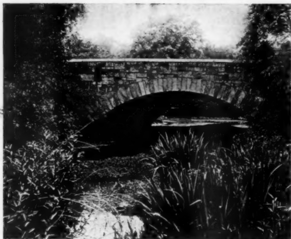
BELLEVUE STREET BRIDGE
