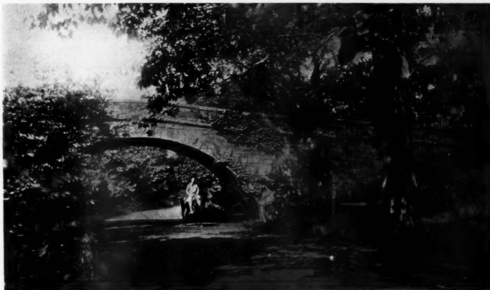
BERNIER STREET BRIDGE OVER BRIDLE PATH
