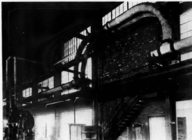
Showing the location of the steam lines that extend around the Steam Forge Shop, and the method of looping these lines to care for expansion and contraction. Under the steam lines is the air line.
