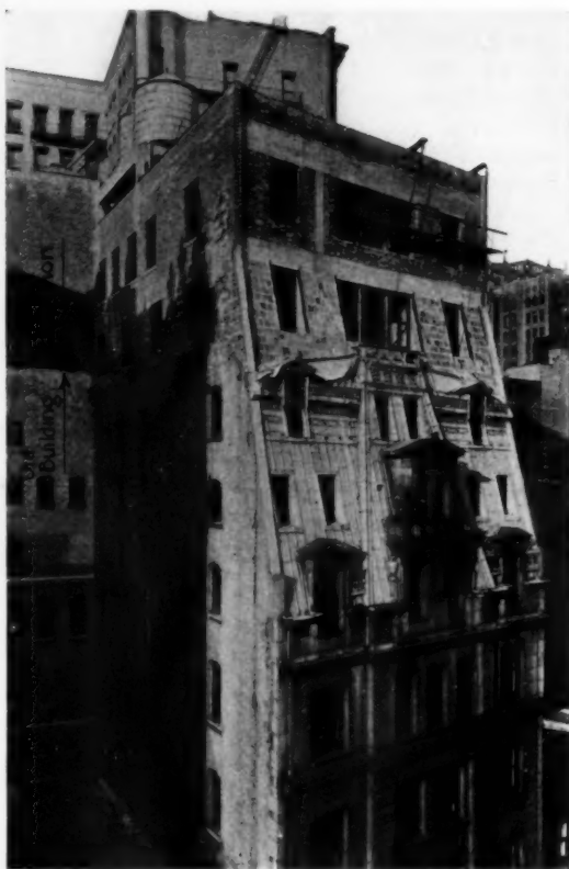
UPPER PART BEAVER STREET ELEVATION, WELLES BUILDING, NEW YORK CITY. ADDITION TO ORIGINAL BUILDING CLEARLY SHOWN
