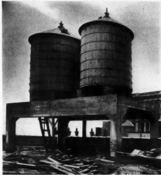
REINFORCED CONCRETE STRUCTURE, SUPPORTING TANKS. NOTE CONCRETE GUSSETS AFFORDING ADDED RIGIDITY
