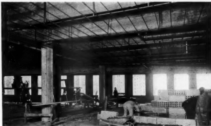
INTERIOR OF ELEVENTH STORY LOOKING TOWARD BROADWAY FRONT. LOWER PART OF CONCRETE GIRDER CAN BE SEEN ALONG FRONT WALL PROJECTING BELOW CEILING LINE.
