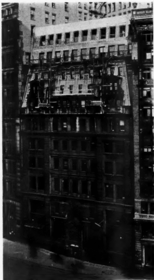
ELEVATION OF BROADWAY FRONT, WELLES BUILDING, NEW YORK CITY, SHOWING WORK ON ADDITIONAL STORIES IN PROGRESS
