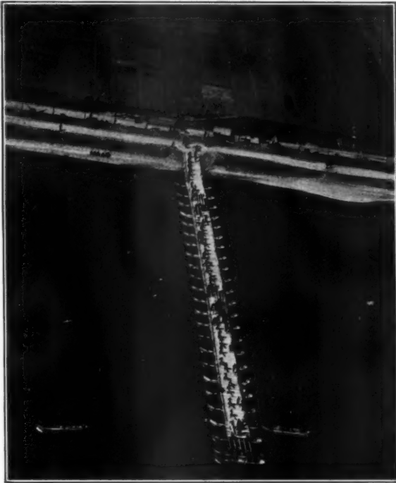
AMERICAN ARMY ENGINEERS CONSTRUCTING RHINE PONTON BRIDGE, PHOTOGRAPHED FROM AIRPLANE
