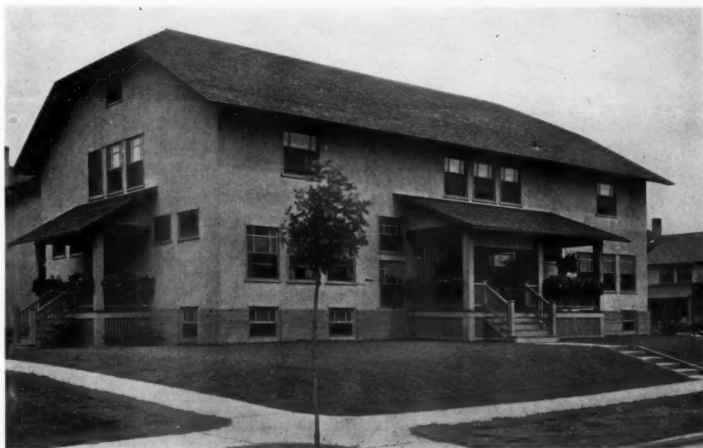
NEIGHBORHOOD CLUB, MORGAN PARK, MINN. DEAN & DEAN, ARCHITECTS
