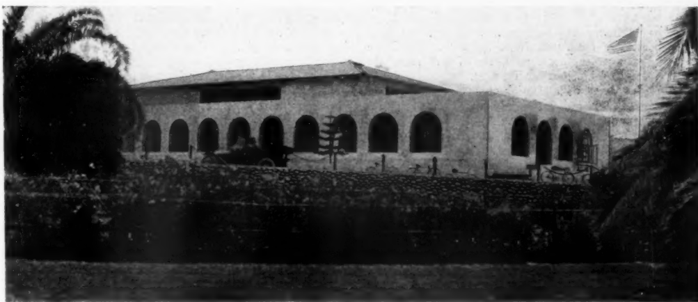
COMMUNITY HOUSE, SAN DIEGO, CAL.
