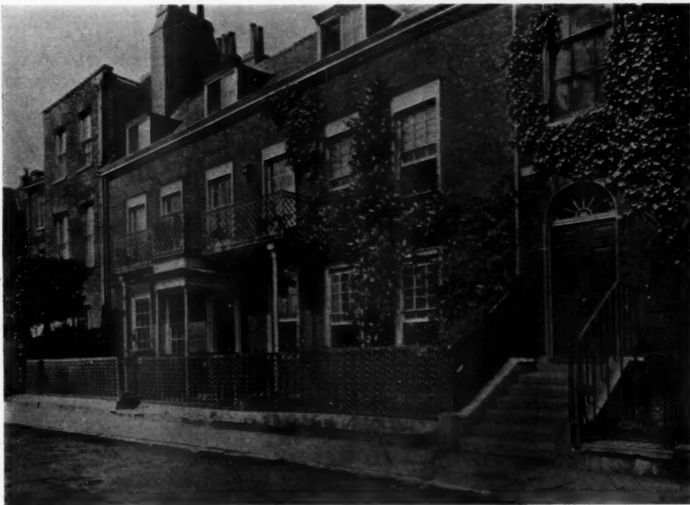
STRAWBERRY HOUSE, THE MALL, CHISWICK
