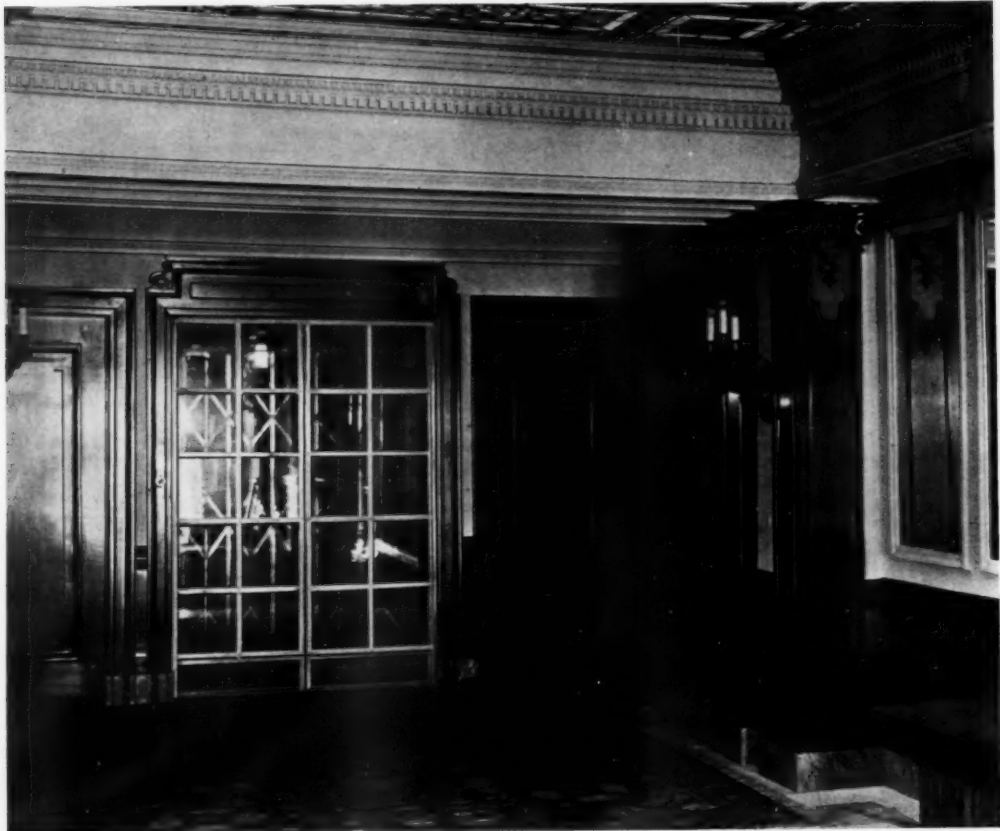
IN THE APARTMENT HOUSE THIS TYPE OF ELEVATOR COMBINES EFFICIENCY AND ECONOMY. NOTE THAT CAR GATE AND SHAFT DOOR ARE CLOSED AND CAR IS READY TO RESPOND TO A CALL FROM ANY FLOOR, OR DOOR MAY BE OPENED TO RECEIVE A PASSENGER ENTERING MAIN HALL
