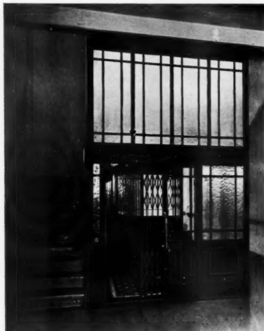
A HOSPITAL INSTALLATION. CAR GATE AND SHAFT DOOR HAVE BEEN LEFT OPEN TO HOLD CAR AT LANDING FOR PATIENT
