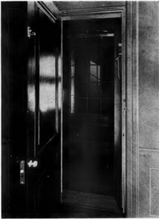
THE SAFETY DOOR LOCK IS HERE SHOWN IN PLACE. NOT UNTIL THE SWINGING DOOR IS CLOSED CAN THE CAR BE OPERATED
